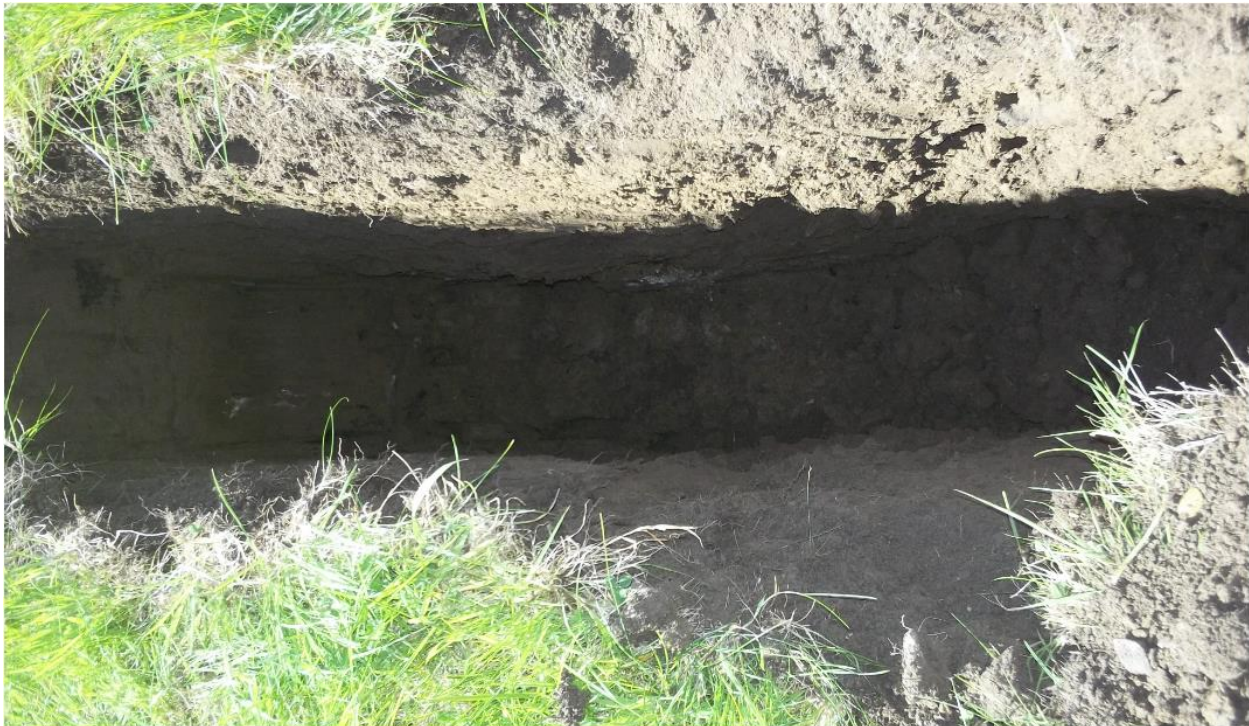
Test Pit before water added – Depth 0.8m
