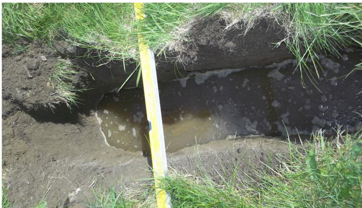
Pit during test
