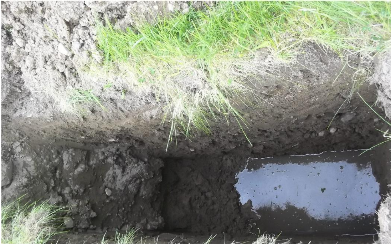
Trial Pit – Depth 2.0m– water settled at 1.5 bgl
