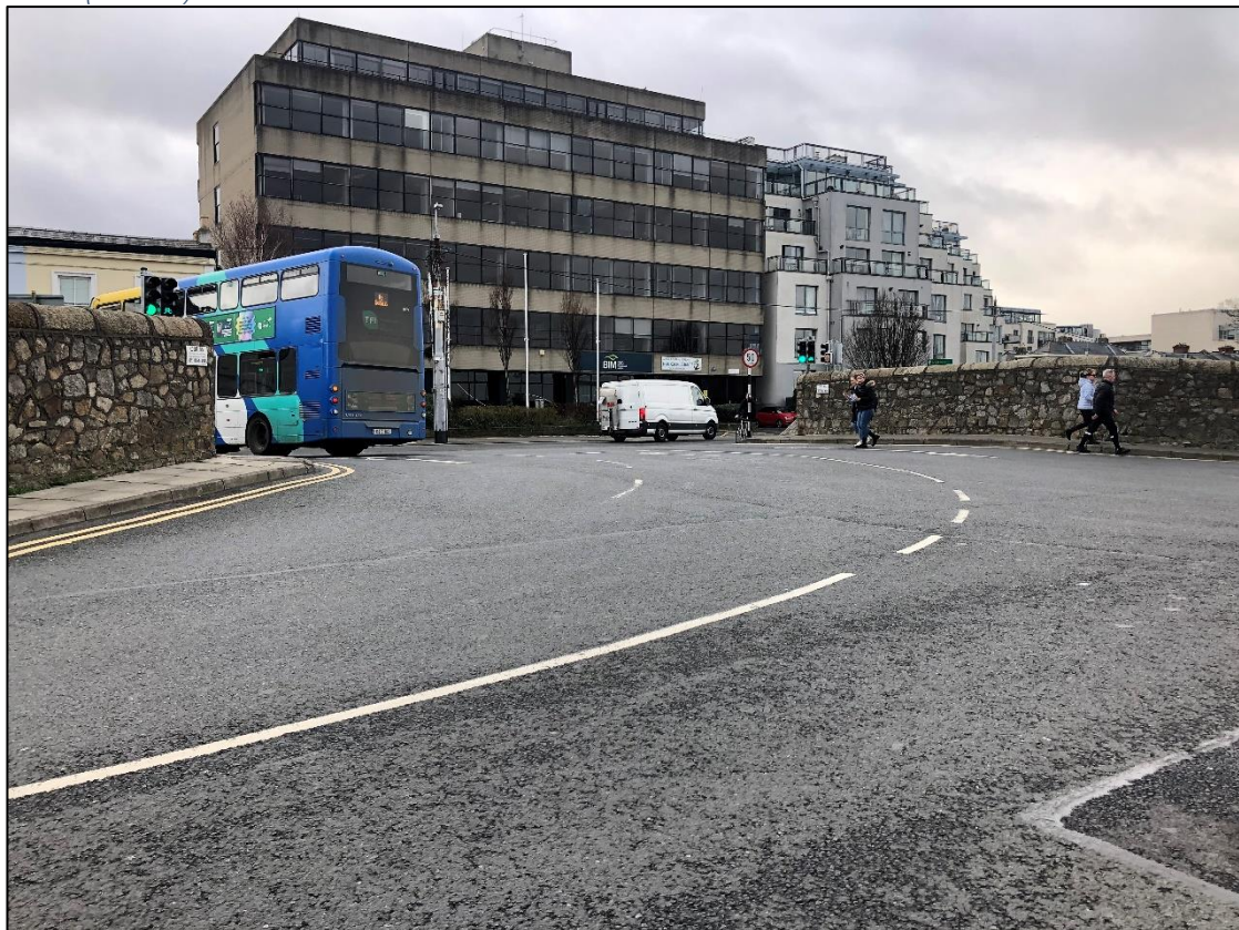
Plate 2-2 Buildings and Artificial Surfaces (BL3) (Road, Pathways, Cycle Lane, Concrete wall, Public Buildings) at Coal Quay Bridge (Section B) to the south of the works area.
