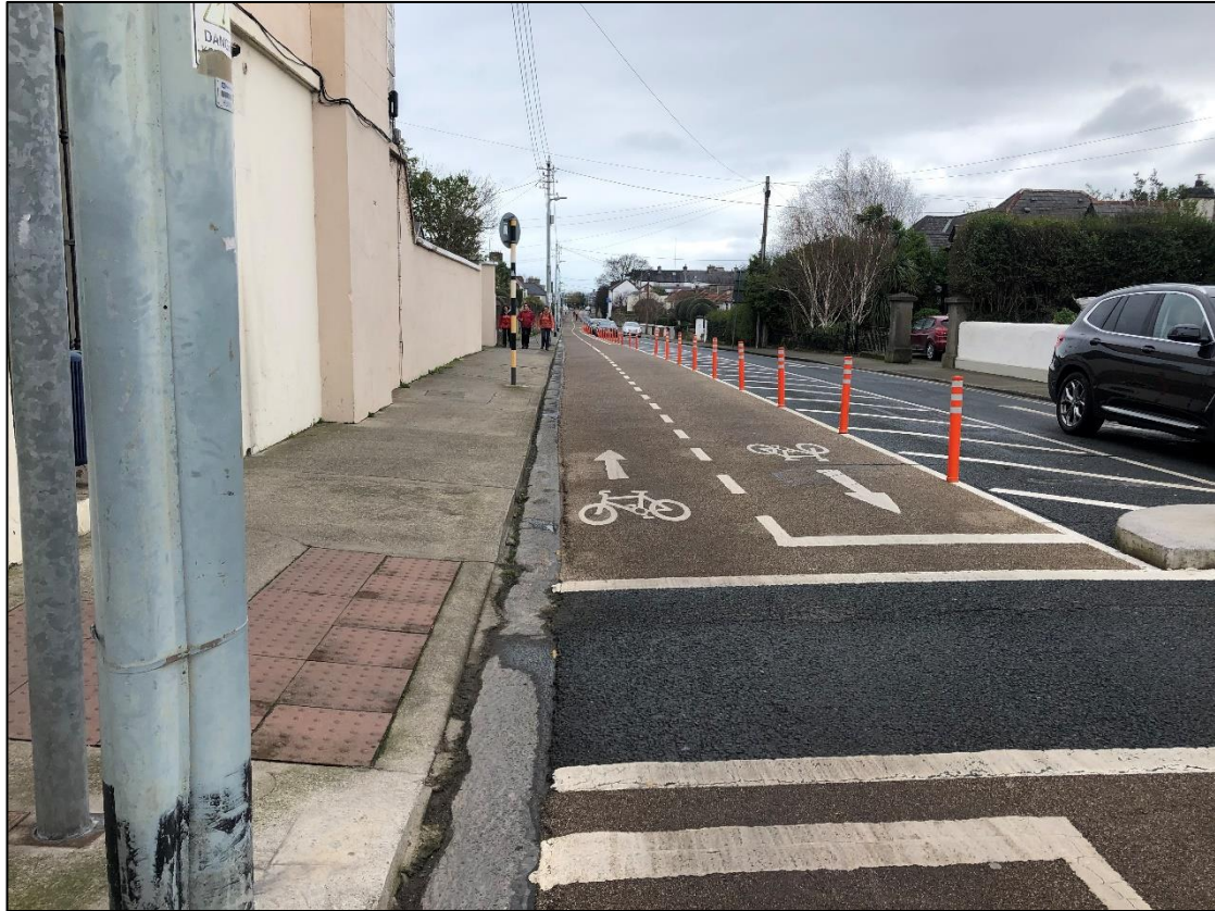
Plate 2-1 Buildings and Artificial Surfaces (BL3) (Road, Pathways, Cycle Lane, Concrete wall, Residential dwellings) at Seapoint Avenue (Section A) to the south of the works area.
