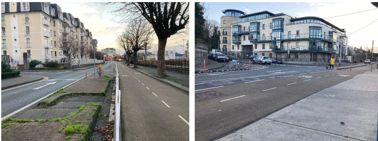
Figure 35 Old Dunleary Road (left) and junction with Cumberland St (right)
