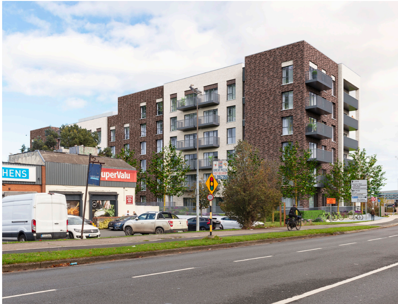
Image 26: View from west along Blackthorn Drive; Balally Shopping Centre on the left
