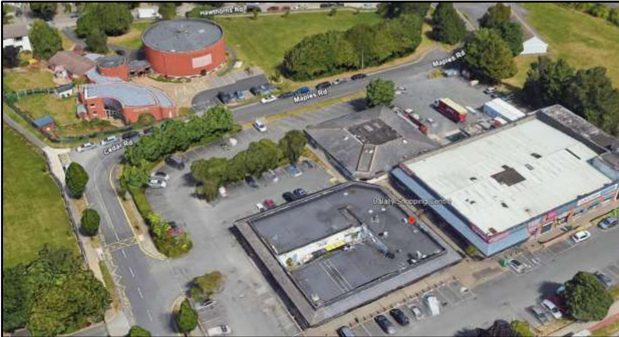
Figure 2.5: Overview of Maples Rd (Source: Google Earth)
