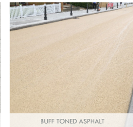
BUFF TONED ASPHALT
