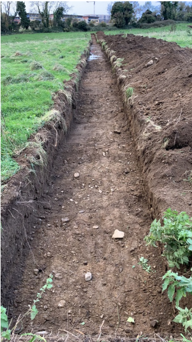
Below: North-facing photograph of TT4
