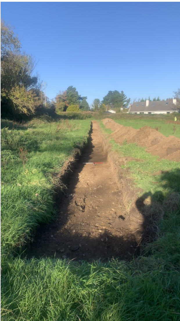
Below: North-facing photograph of TT1
