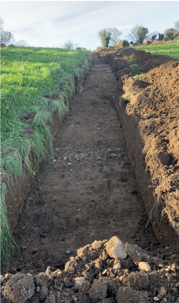
Below: West-facing photo of TT5 showing F12
