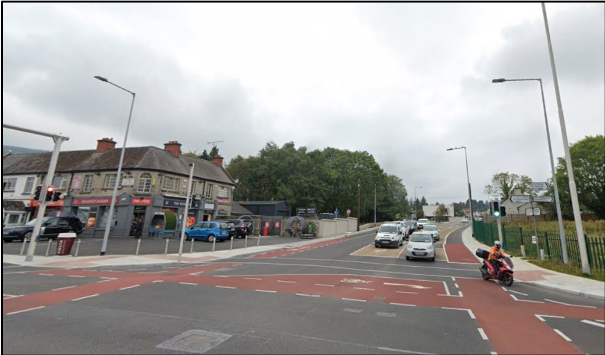
Figure 3.3: Signalised Pedestrian Crossings at Lamb’s Cross Junction, in the Vicinity of the Site (Source: Google Street View)
