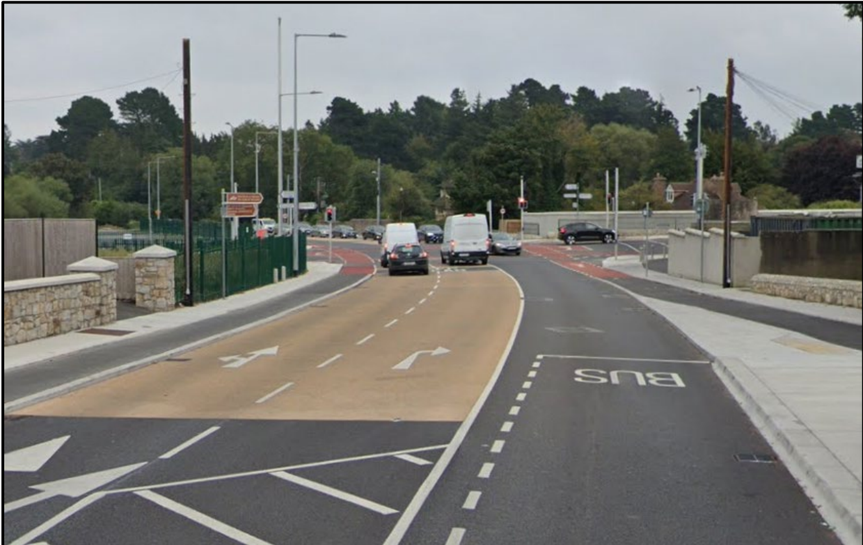
Figure 3.7: Existing Cycle Infrastructure Along Blackglen Road Approaching the Lamb's Cross Junction (Source: Google Street View)
