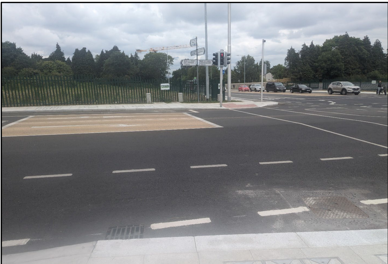
Figure 3.1: View of Lamb's Cross Junction As Someone Approaches From Enniskerry Road (Source: ORS, 17/06/2024)
