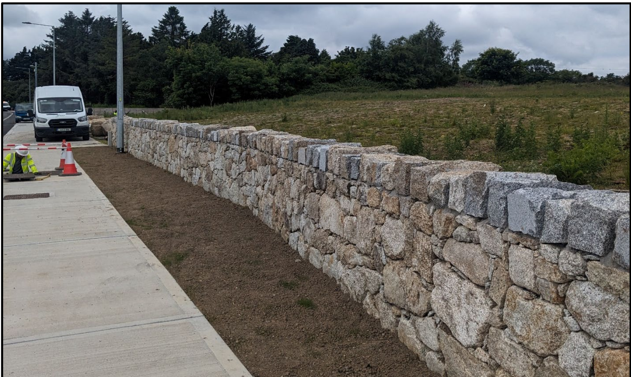
Figure 2.7: View of Existing Boundary Arrangements at the Site Frontage, Along Blackglen Road (Source: ORS, 17/06/2024)
