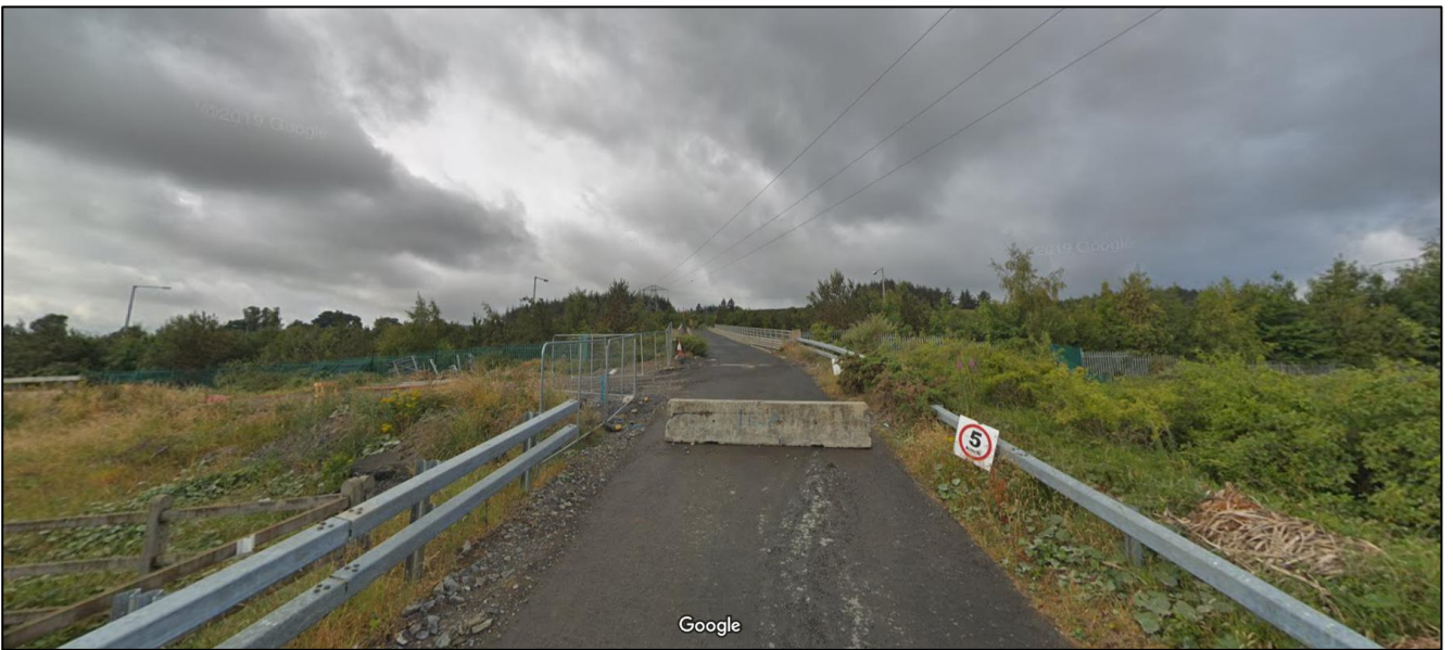
Figure 3-6: Lehaunstown Lane looking at closed bridge over the M50. (Southwestern end of Lehaunstown Lane)
