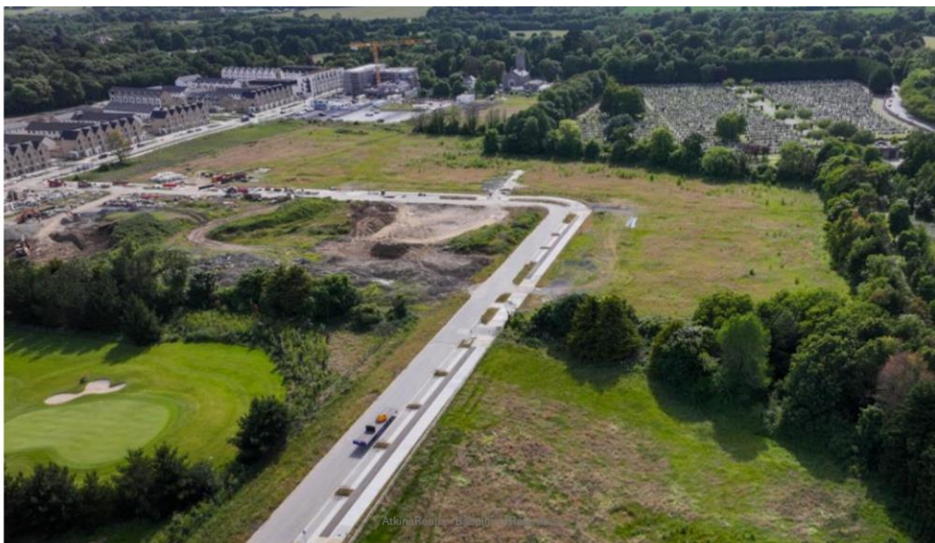
Figure 3-2 - As built Woodbrook Avenue
