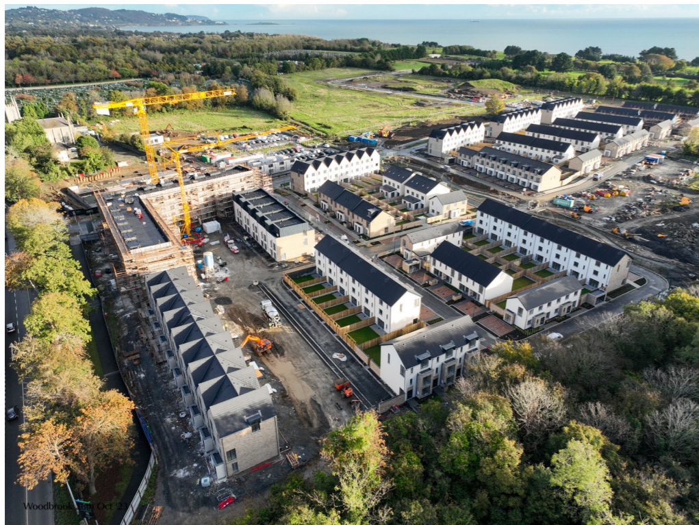
Woodbrook Phase 1: Construction Photograph
