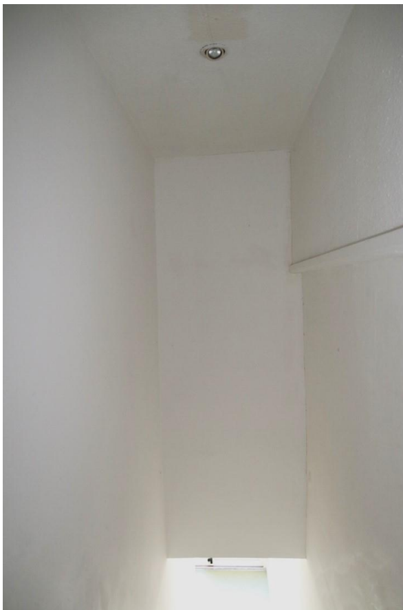
Plate 98: Walls and ceiling over staircase
