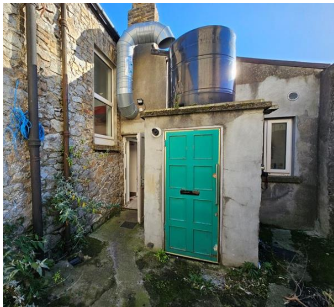
Plate 17: Eastern return and boiler house
