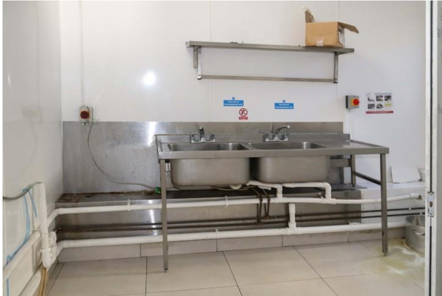
Plate 64: Southern wall of scullery
