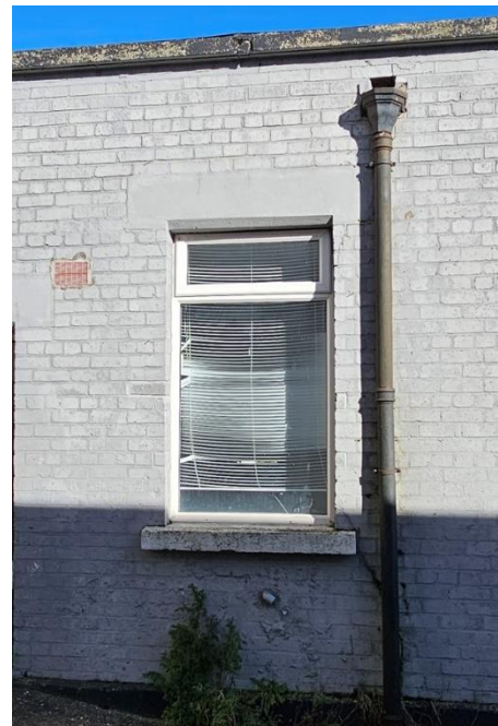
Plate 14: Window in rear extension
