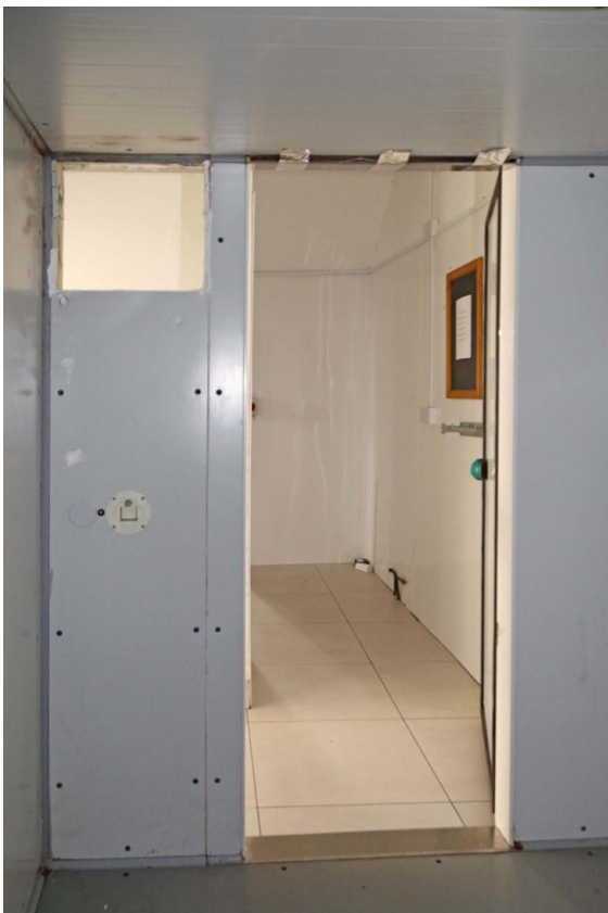
Plate 61: internal face of refrigerator doorway
