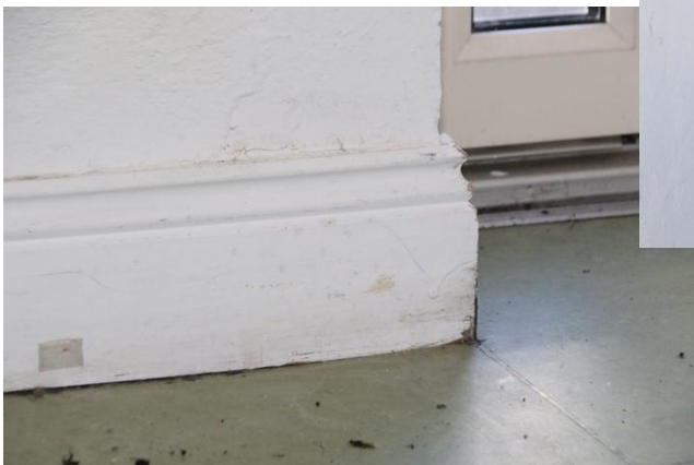
Plate 33: Skirting in entrance hall
