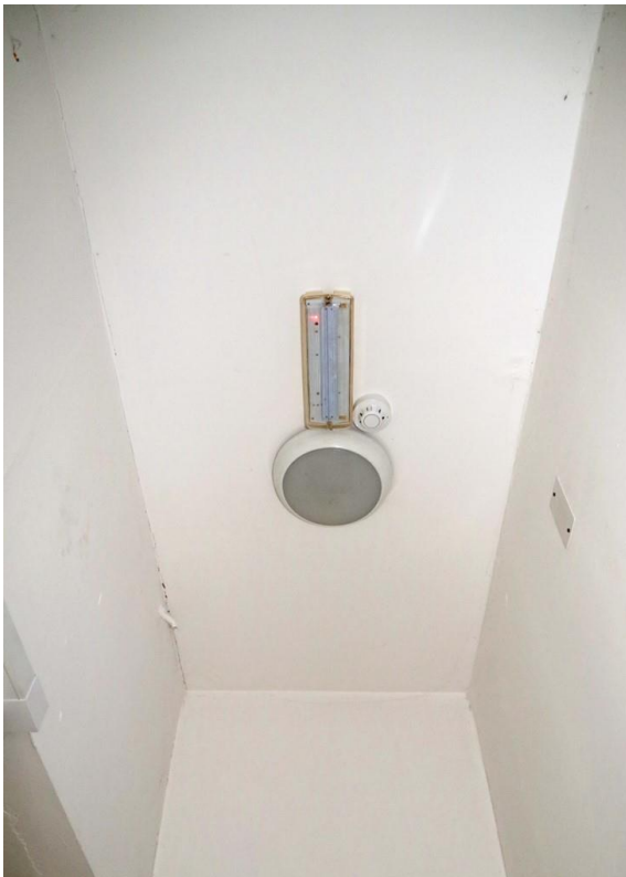
Plate 58: Ceiling in lobby
