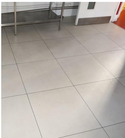
Plate 56: Floor in kitchen
