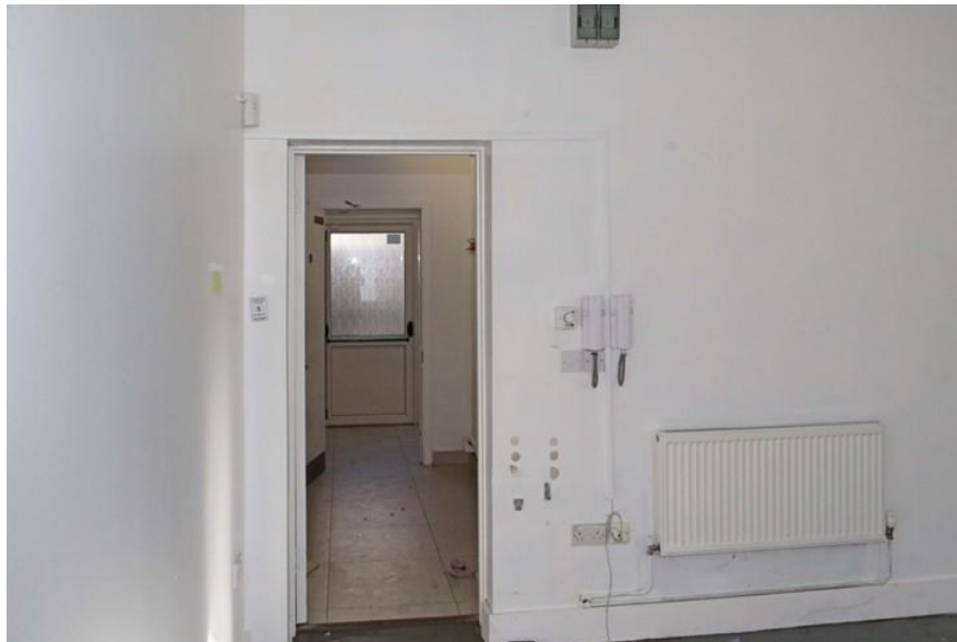
Plate 89: Doorway into office from corridor
