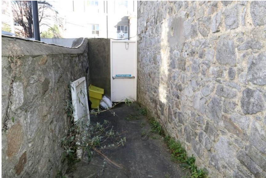
Plate 24: View to front of passageway
