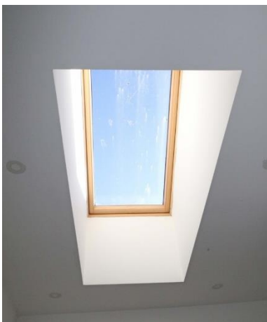
Plate 73: Skylight in lobby
