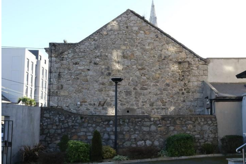
Plate 26: Western gable of building
