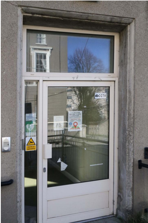
Plate 3: Doorway at western end of facade
