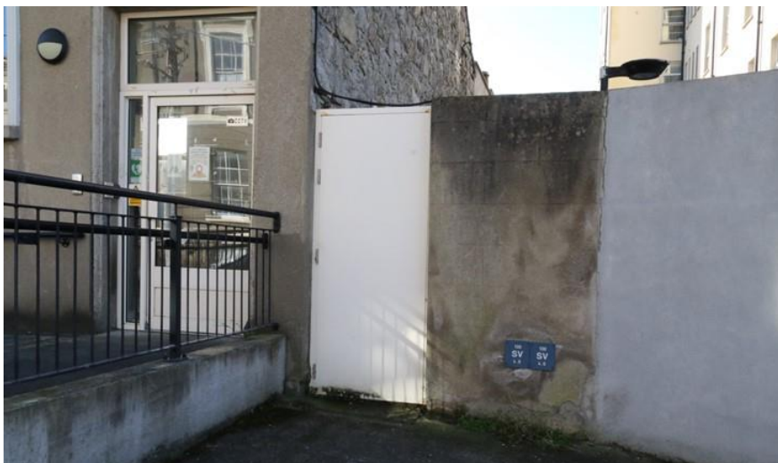
Plate 2: Doorway at western end of building
