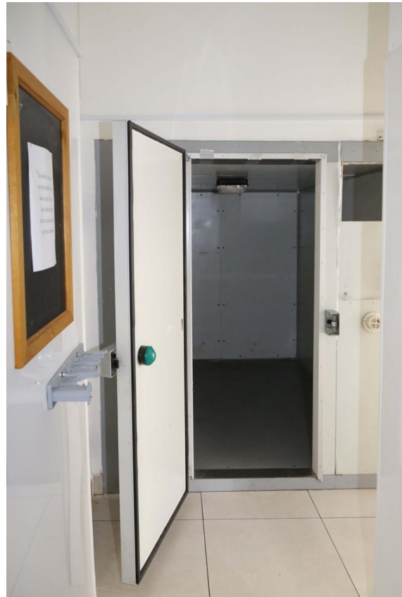
Plate 57: Lobby and refrigerator door
