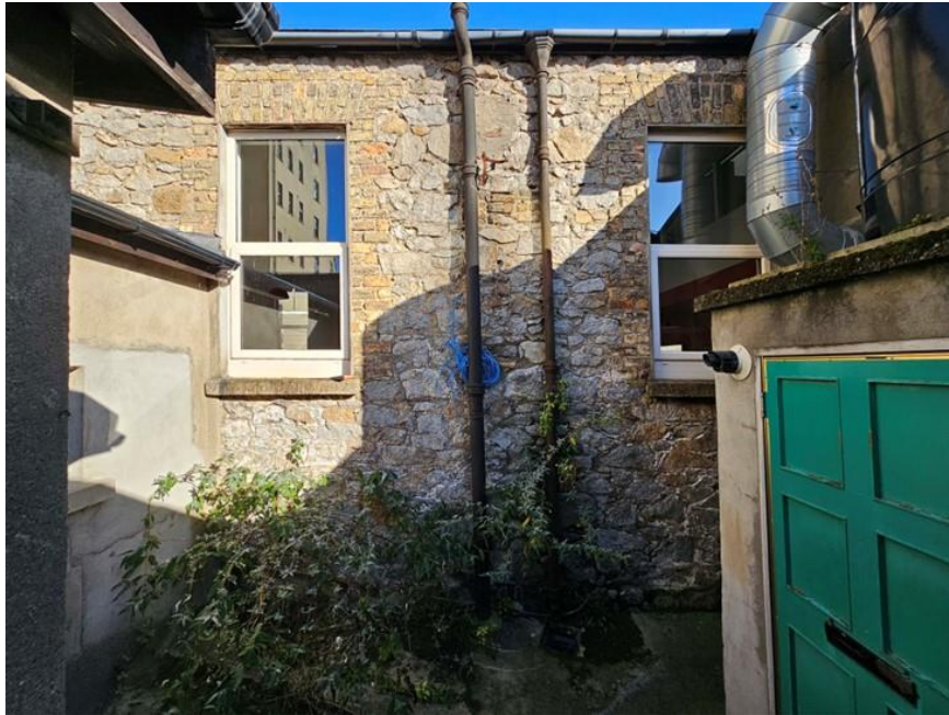
Plate 16: Rear façade of main building
