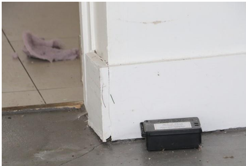
Plate 91: Skirting in office
