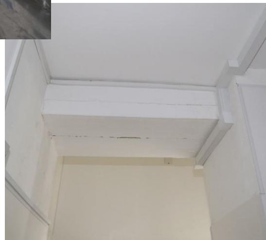
Plate 55: Beam over doorway to scullery
