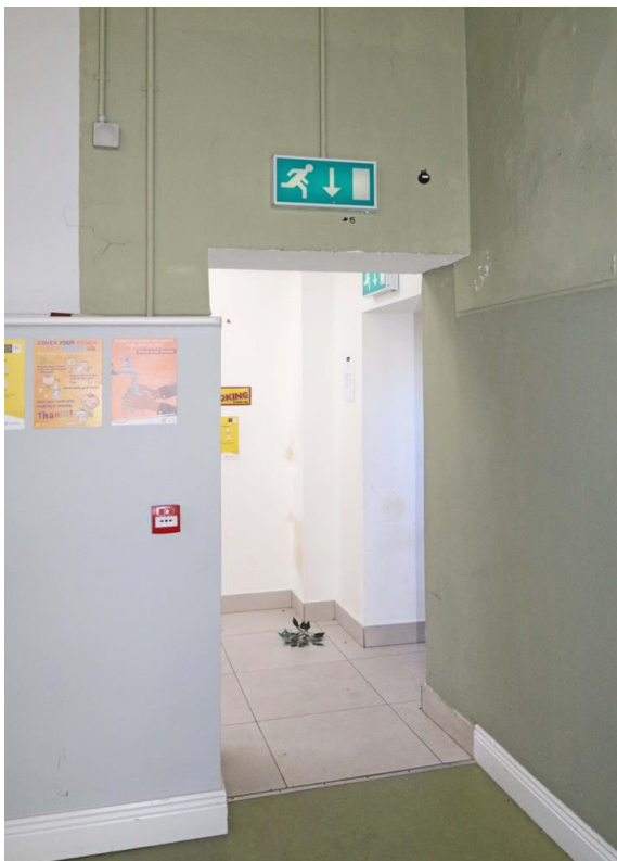
Plate 43: Access to western return
