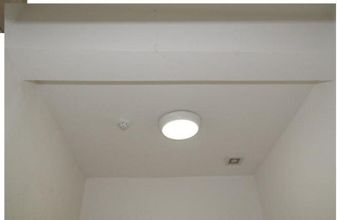
Plate 76: Beam in ceiling
