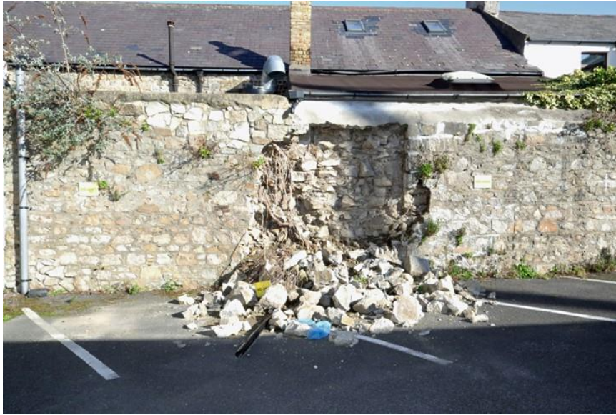
Plate 8: Rear boundary wall, with 10 Eblana Avenue beyond
