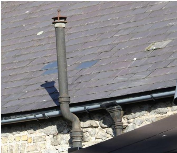
Plate 11: Gutter, downpipe and vent pipe
