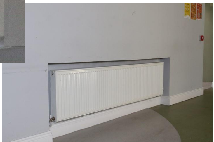
Plate 40: Radiator in rear wall, set back into dry lining
