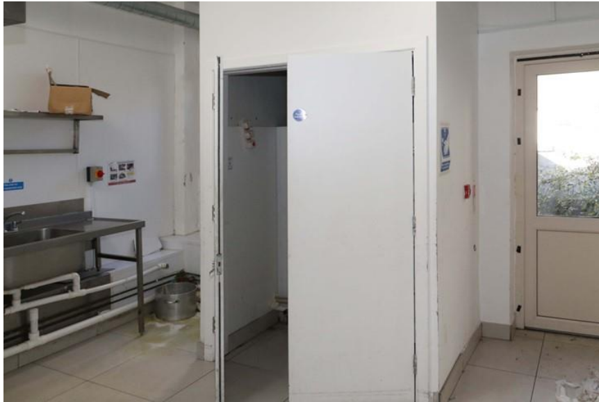
Plate 62: Western wall of scullery
