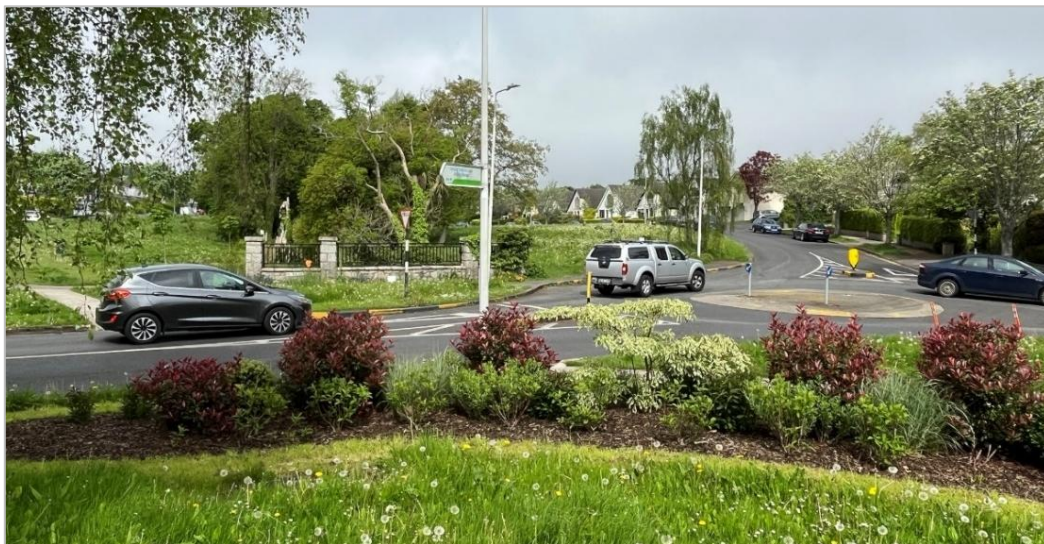
Figure 4-8: View Looking North Towards Glen Lawn Drive / Glen Drive Roundabout
