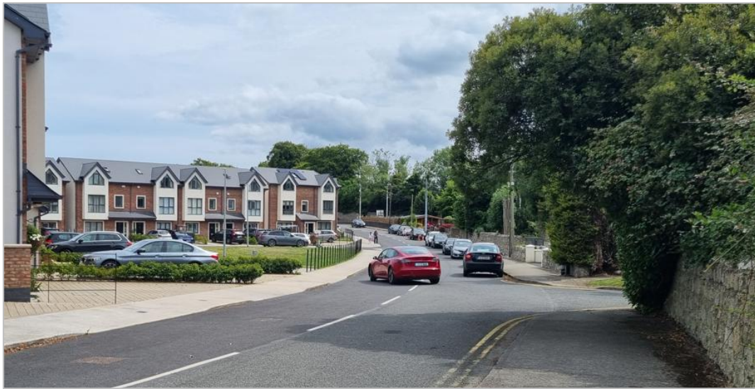
Figure 4-10: View Looking South on Clonkeen Road
