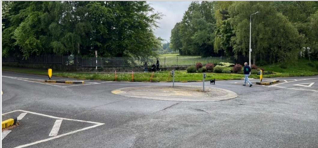
Figure 4-7: Poor Pedestrian Facilities at Glen Lawn Drive / Glen Drive Roundabout
