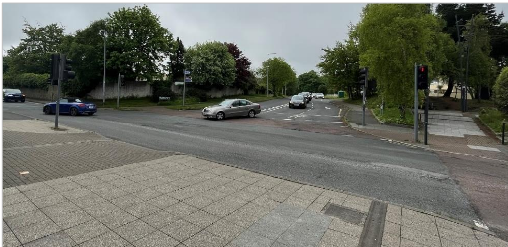
Figure 4-2: View Looking South at the Bray Road / Cornelscourt Hill Road Signalised Junction
