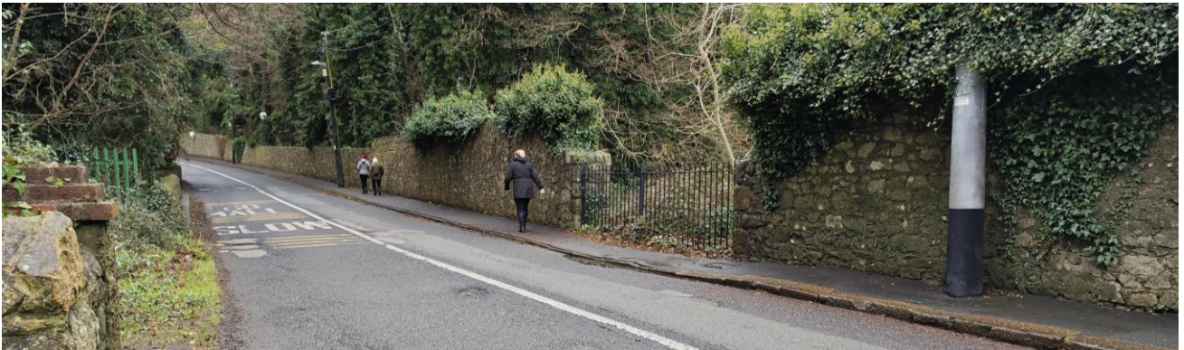
Figure 19: View from Brennanstown Road of the eastern boundary of Cabinteely Park (Source: MDB)
