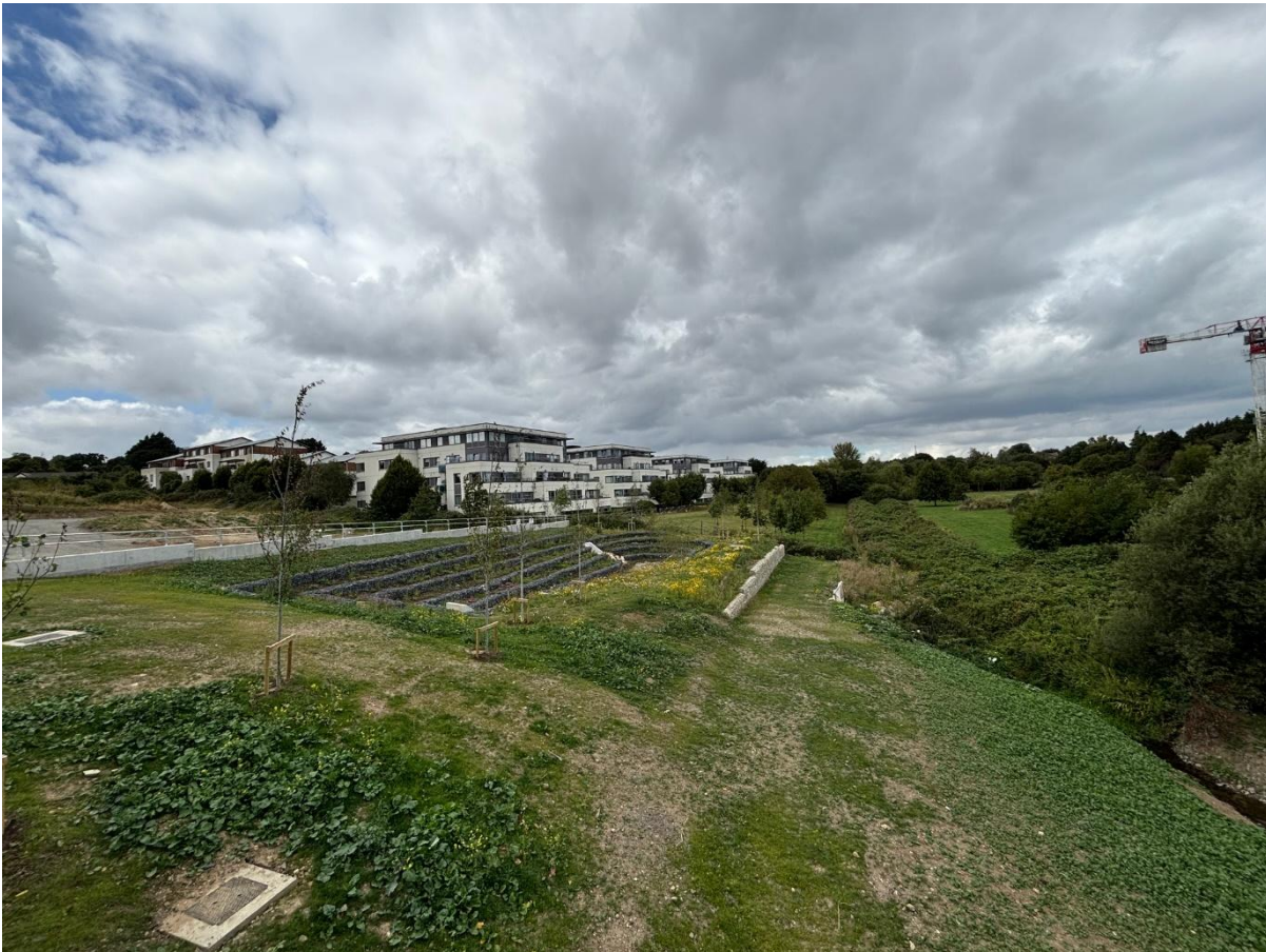
Figure 6: View of Brennanstown Square development (facing north) (Source: MDB)
