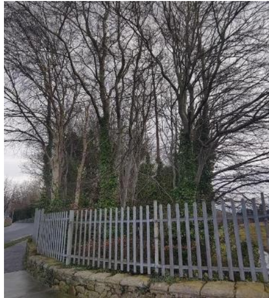
Section of wall which will be removed to facilitate route entrance to the park.
