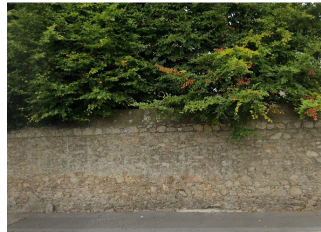
Cabinteely Park Boundary Wall to Old Bray Road.
