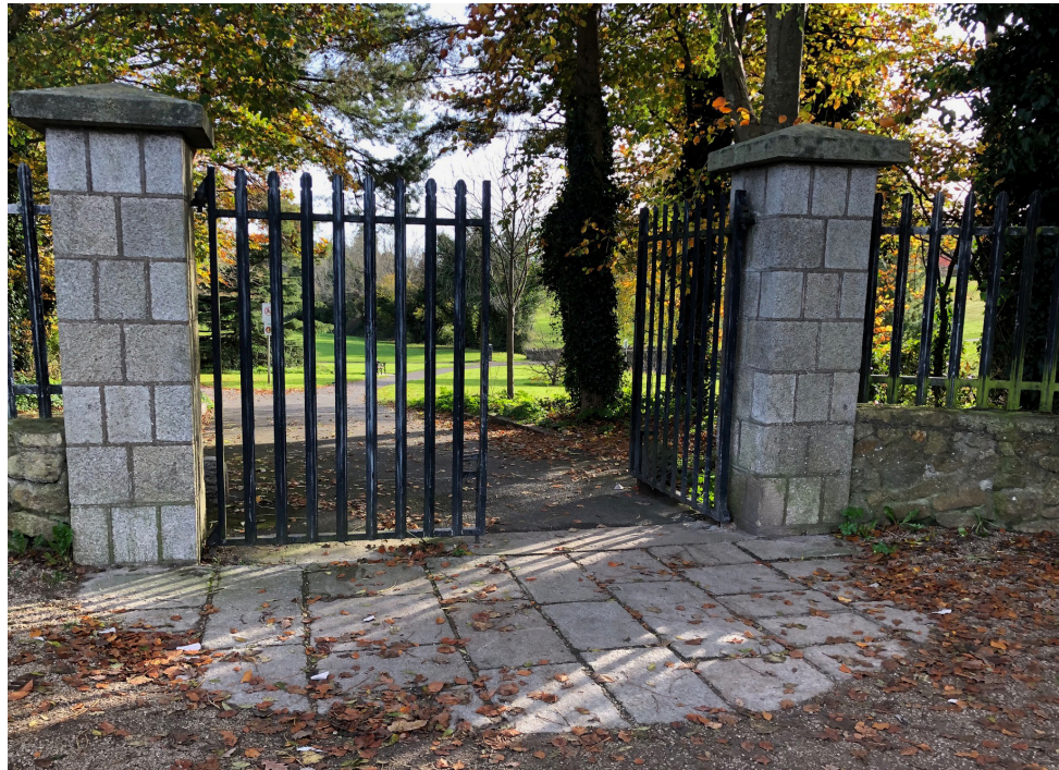
Existing Glen Drive entrance with Granite Pavers.
