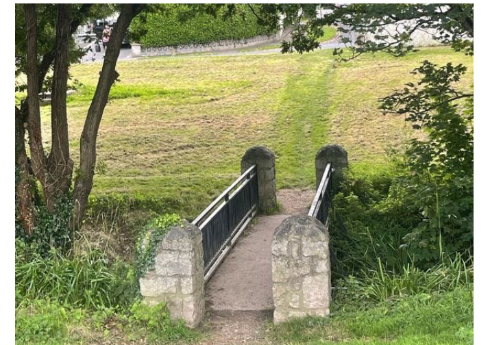
Glen Lawn One of the small bridges over the stream
