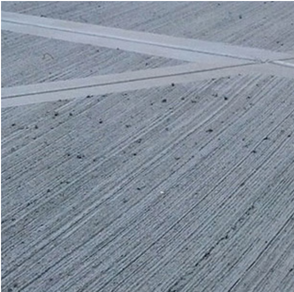
In-situ concrete to foopaths.
