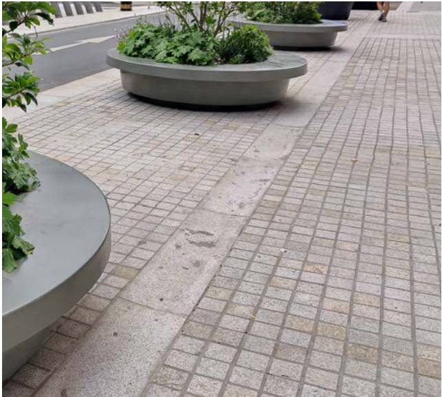
Granite setts to feature locations
