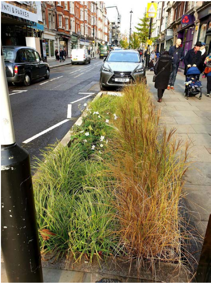
Above: example of Planted Rain Garden, London.
