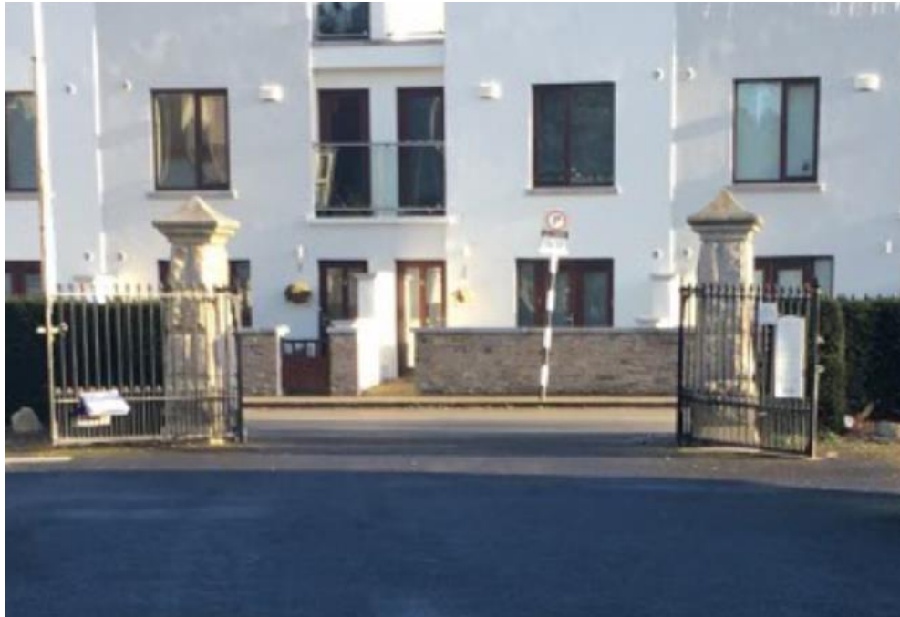
Figure 6-24: Existing Piers at Southern Vehicle Entrance to Cemetery
