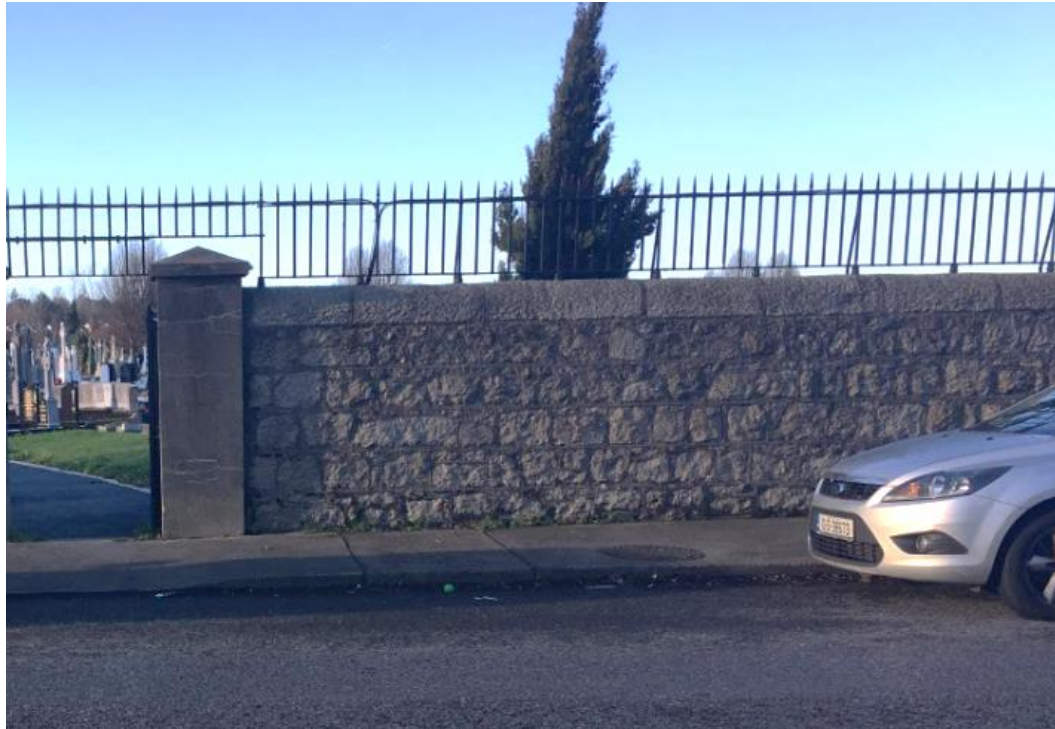
Figure 6-19: Existing Boundary Wall and Railings at Deansgrange Cemetery
