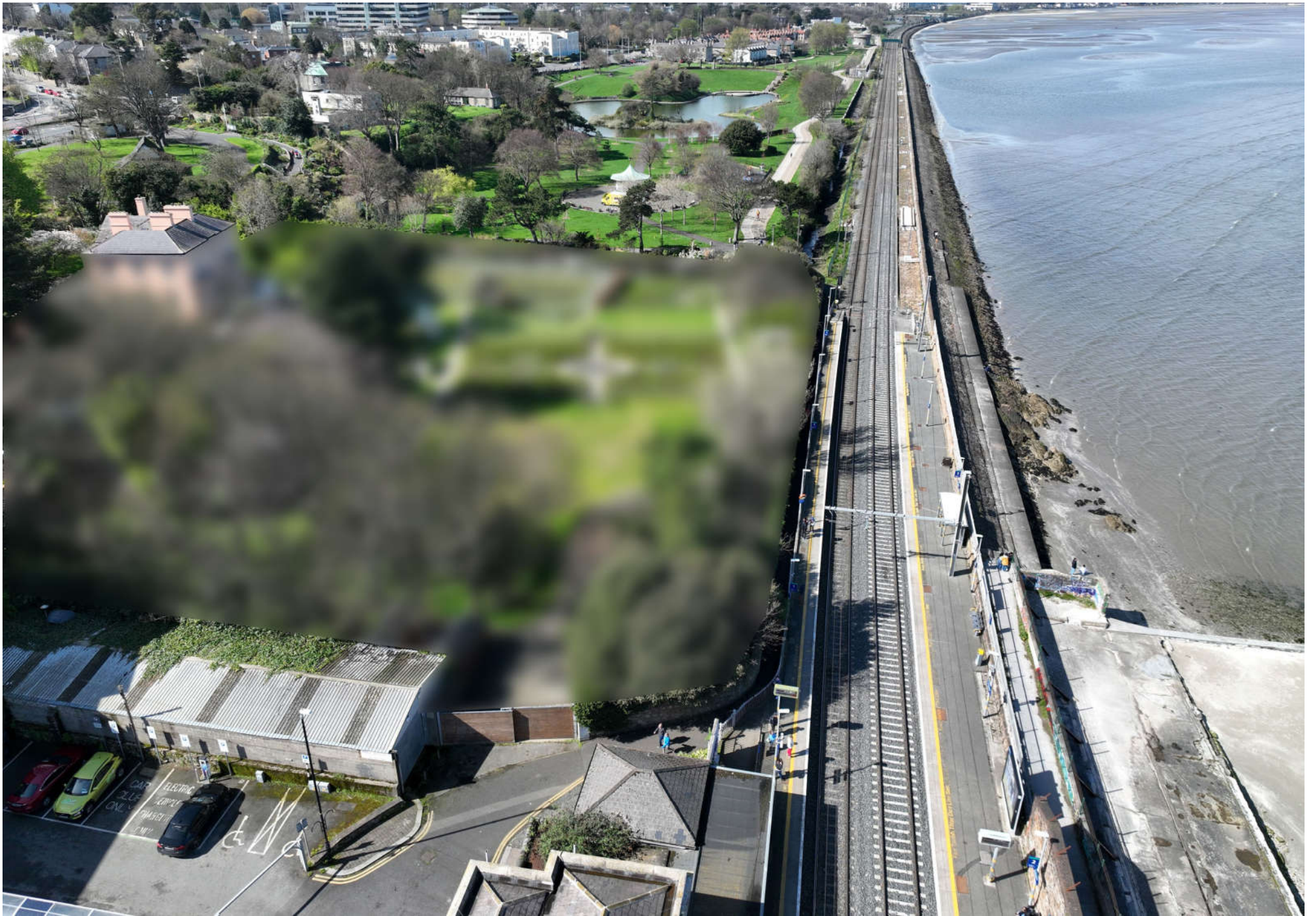
View 2 – Northbound Elevated View Existing
