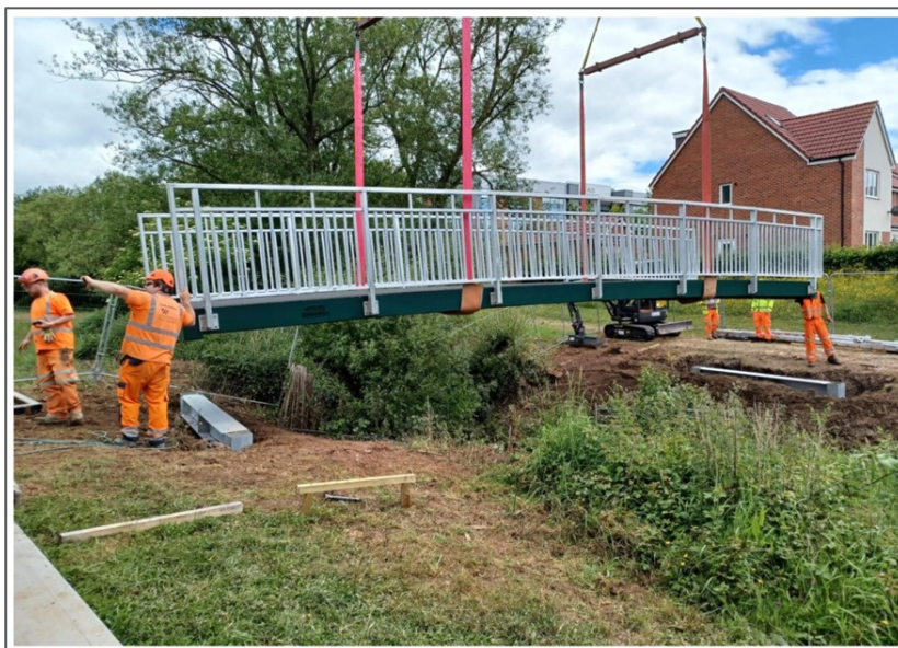
Figure 1-5 - Example of prefabricated bridge unit.
