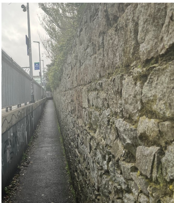
Figure 3-4 – Existing Deepwell House Boundary Wall
