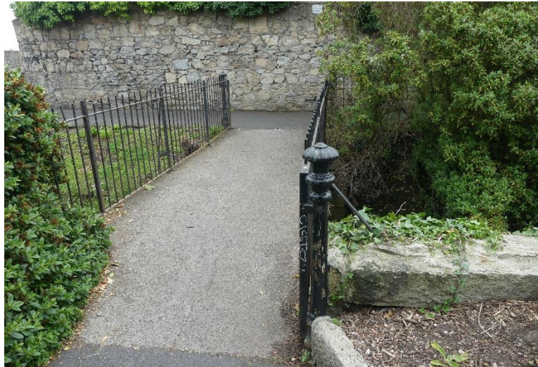
10 View from Park looking East with cast iron post on the right
