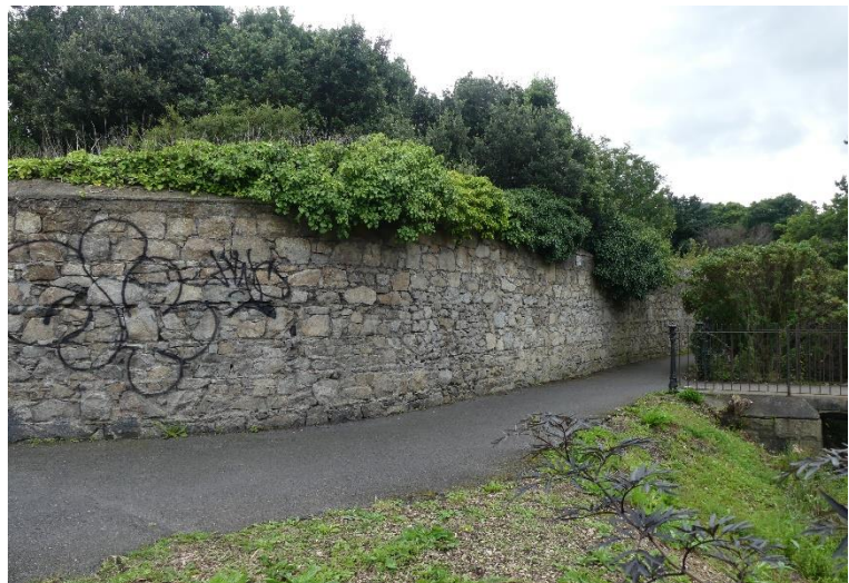
5 View of curved corner
