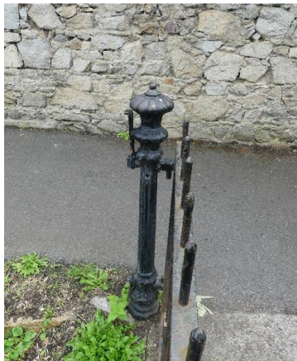
6 Detail of metal post looking east from bridge
