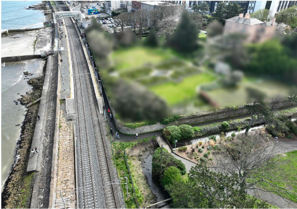
View 1 – Southbound Elevated View Existing
