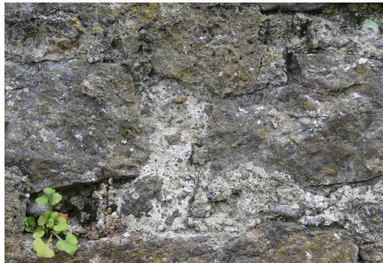
4 Lime mortar detail
