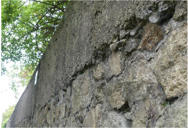
2 Interface between cast concrete elements and original wall
