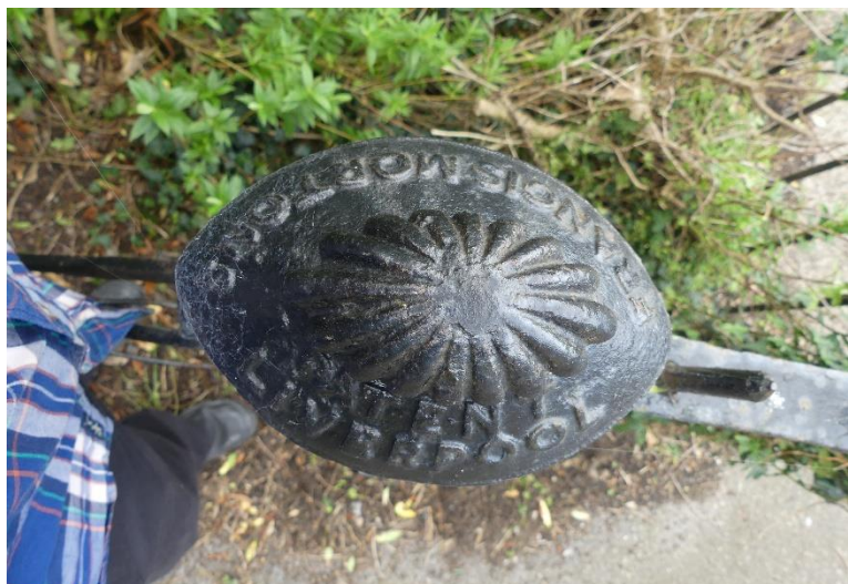
8 Top of cast iron post detail
