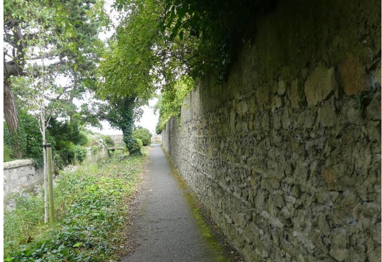
3 View towards Blackrock Park Bridge
