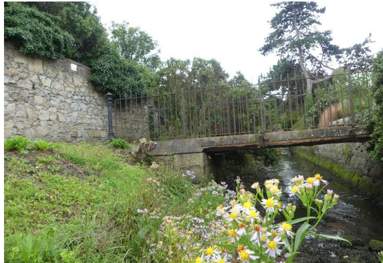
1 View of bridge with Deepwell Boundary wall on the left
