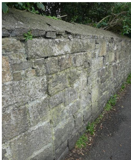
3 View of lintol and stone infill below
