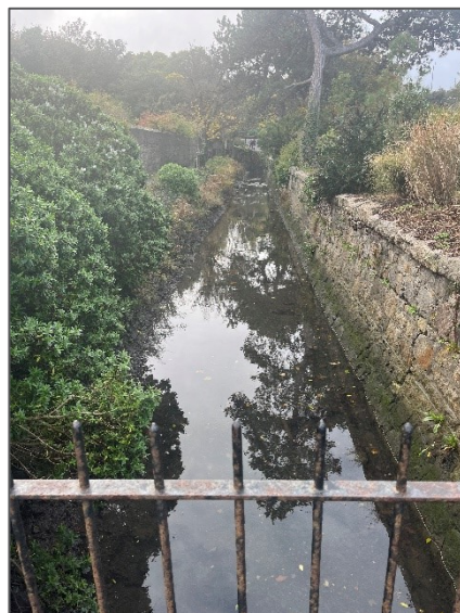
Plate 3-4 Canalised Priory Stream.
