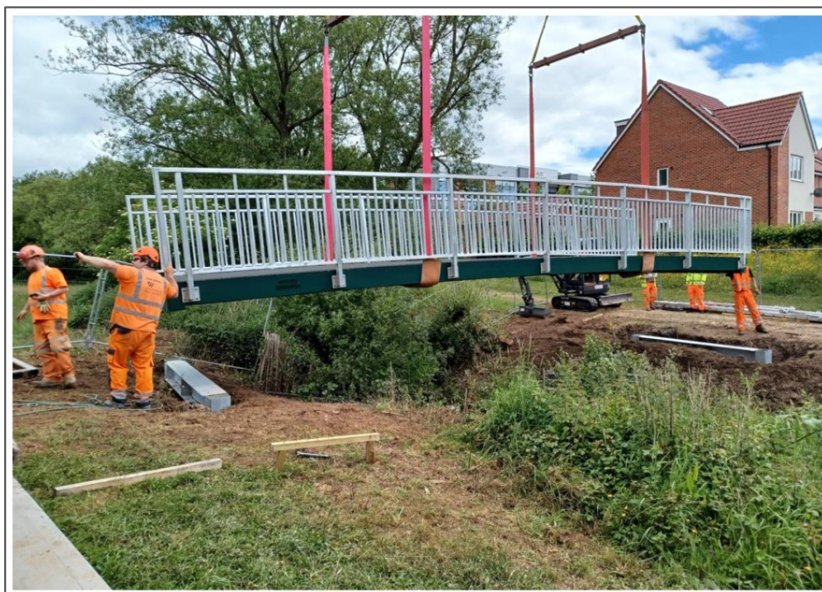
Figure 1-5 - Example of prefabricated bridge unit.
