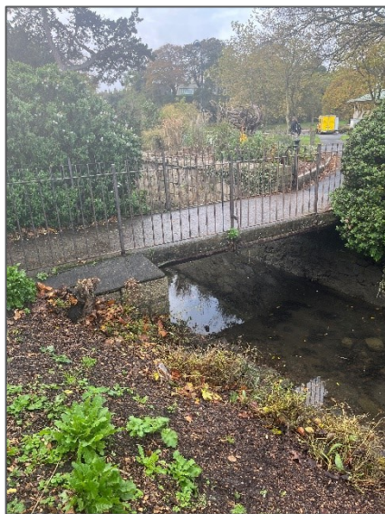
Plate 3-3 Priory Stream with bridge.
