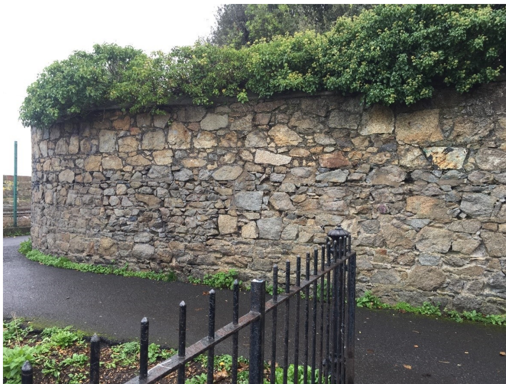
Figure 4-6 – Existing Deepwell House Boundary Wall
