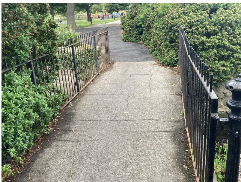
Figure 3-2 – Existing Blackrock Park Bridge over Priory Stream
