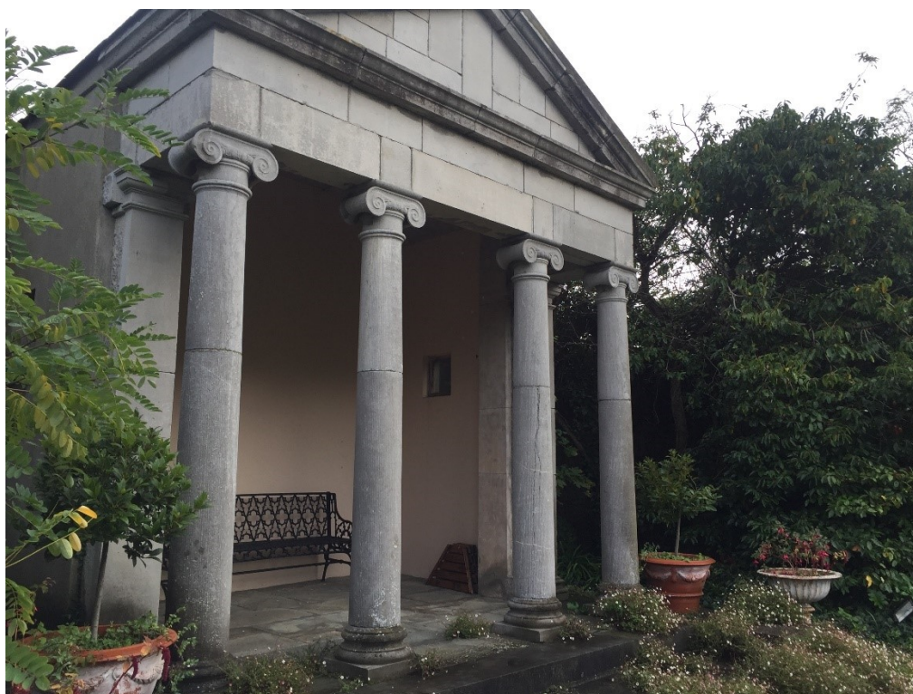
Figure 4-7 – Existing Single Storey Grecian folly
