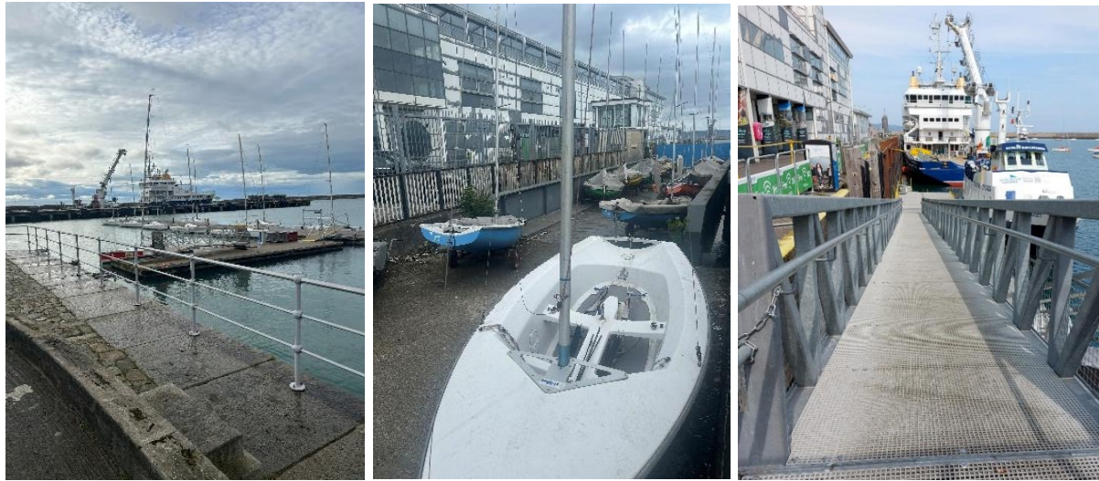
Figure 5, 6 & 7. Photos from St. Michael's Pier
