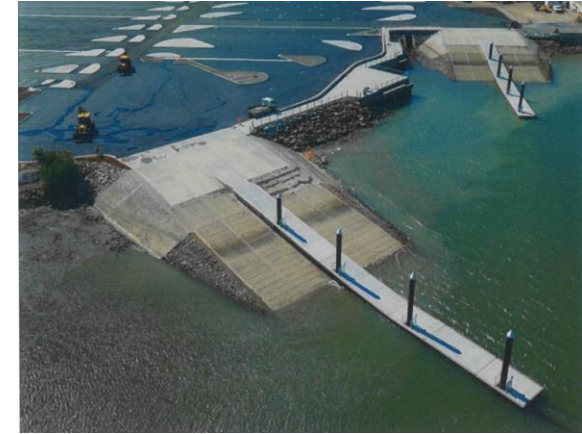
Townsville Slipway, Australia
