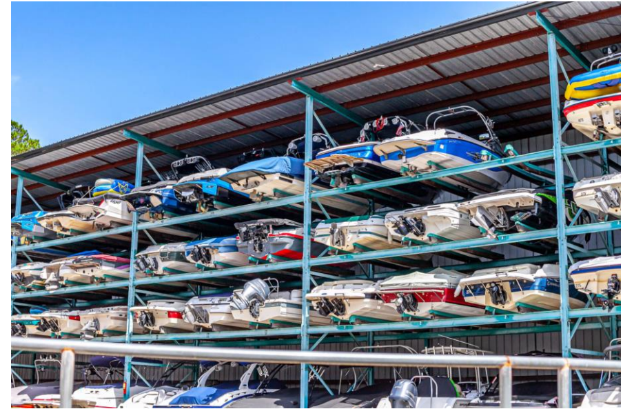
Dry Stack Boat Storage, Lake Allatoona, Georgia, USA
