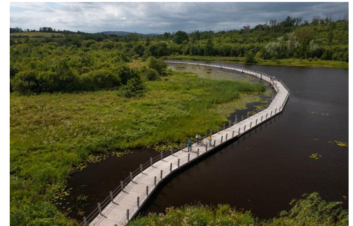
Floating boardwalk, Drumshanbo, Leitrim
