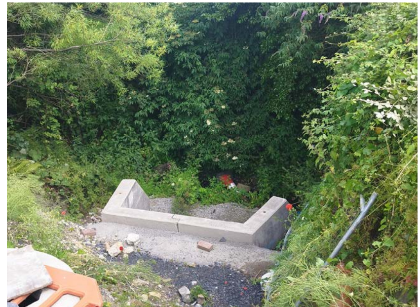
Plate 8: Stream and modern construction on north side of Hillcrest Road.
