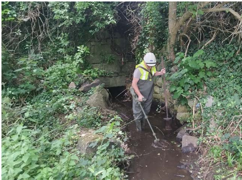
Plate 3: Metal detection in progress looking north.
