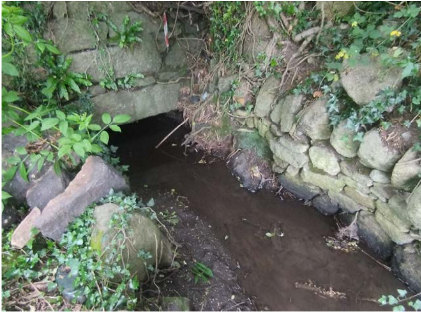
Plate 5: Detail of culvert underneath Hillcrest Road looking northeast.
