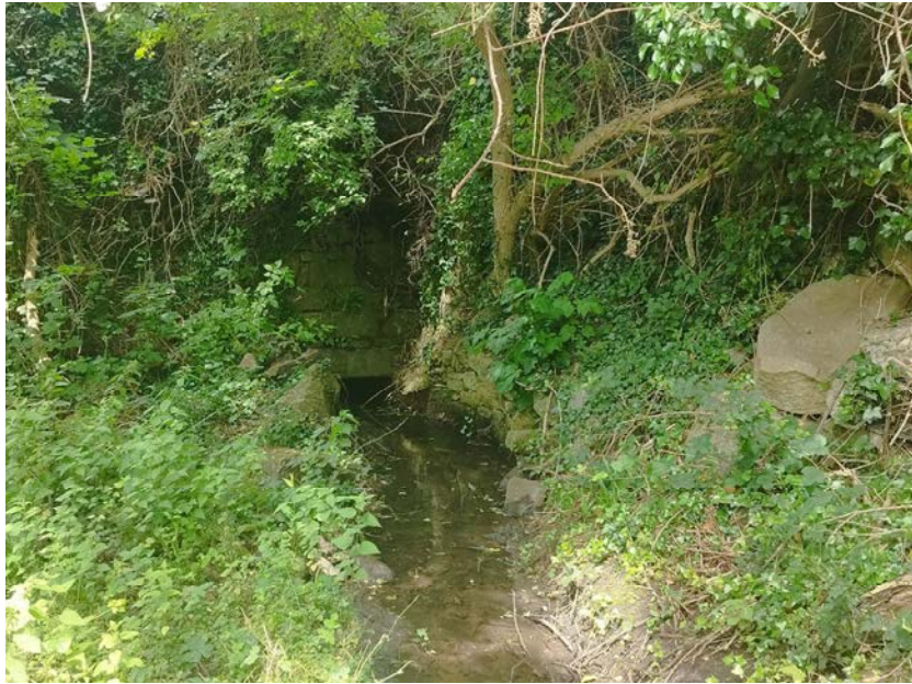
Plate 1: Culvert and stream under Hillcrest Road looking north.
