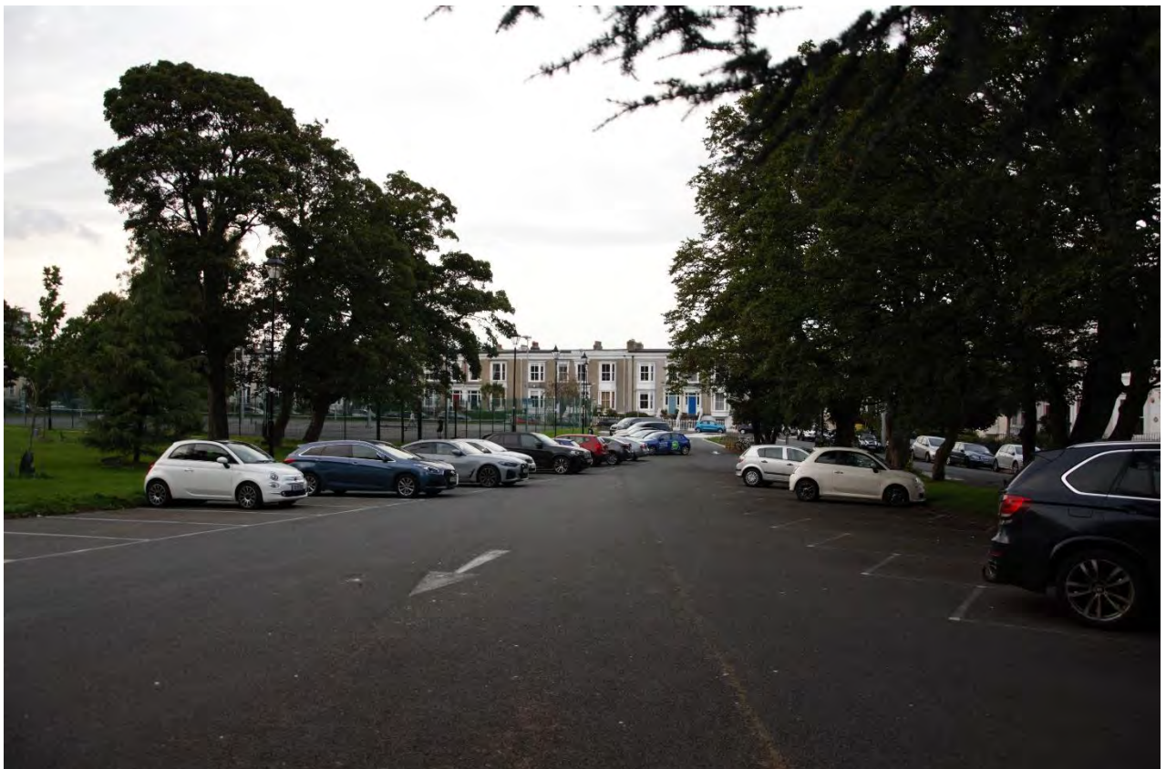
Plate 6: East carpark – looking north.
