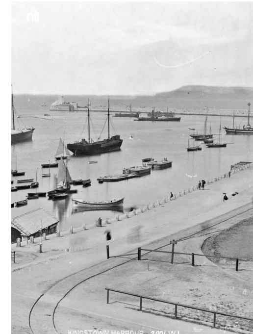
When completed, Dun Laoghaire Harbour became the largest manmade harbour in the world
