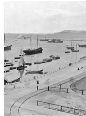
When completed, Dun Laoghaire Harbour became the largest manmade harbour in the world.
