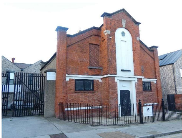
Fig.2: Former Wash House, Kelly’s Avenue.
