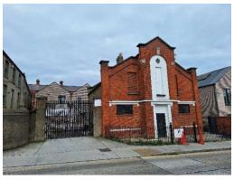
Existing front elevation of Wash House to be restored with windows inserted in blocked-up original opes. Courtyard to be landscaped with pergola overhead between buildings.
