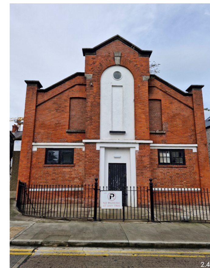
2.46 The former Wash-house and Laundry with railings and gates creating a small entrance court to the street
