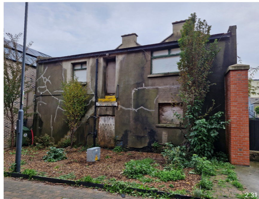
2.30 Eastern façade of former hotel on Kelly's Place behind roughcast concrete walls and railings.
