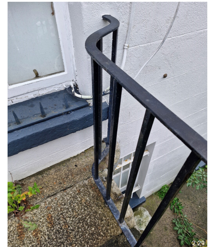
2.28 Curved cut-stone closer to steps and cast- and wrought-iron handrail detail at the entrance. 2.29 Flight of granite steps from Georges Place approaching the entrance and reception room window.
