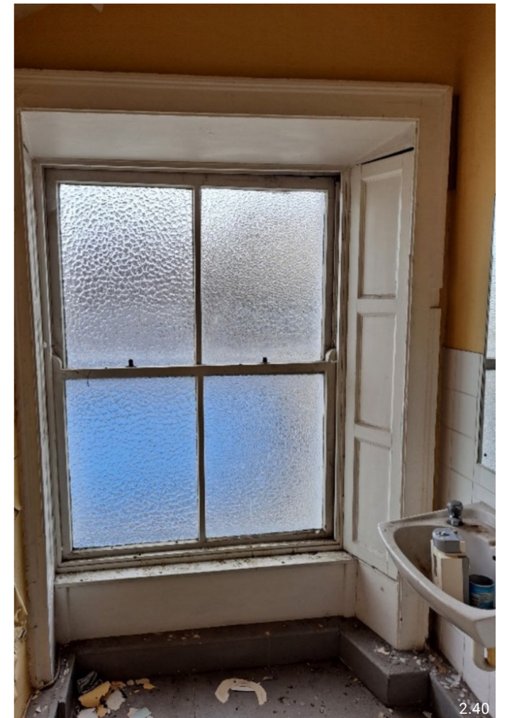
2.38 Moulded timber mantelpiece with later tiled surround in ground floor reception room. 2.39 Doorways to bedroom at first floor level in western bay. 2.40 Two-over-two sash window and panelled shutter boxes in bathroom at first floor level in eastern bay.
