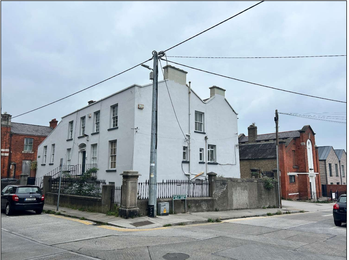
Figure 3.5: Building to be demolished
