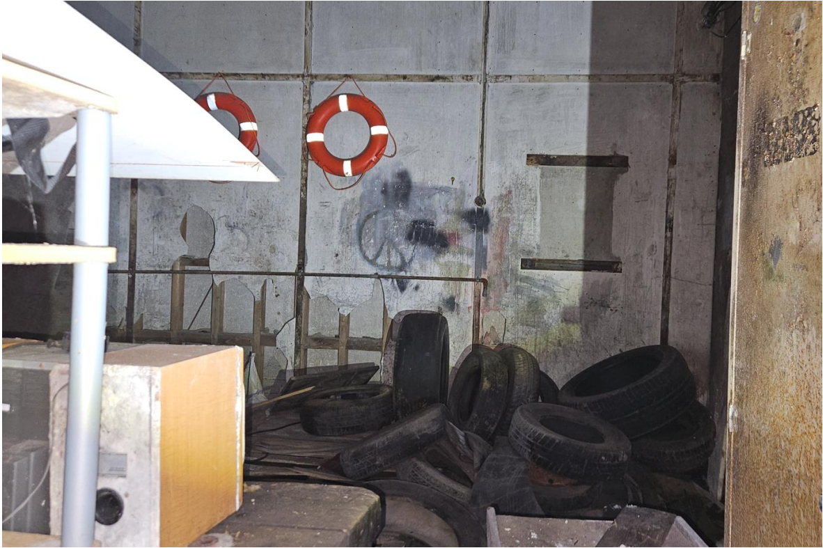
Photo 7. Internal floor of extension (Ground floor)
