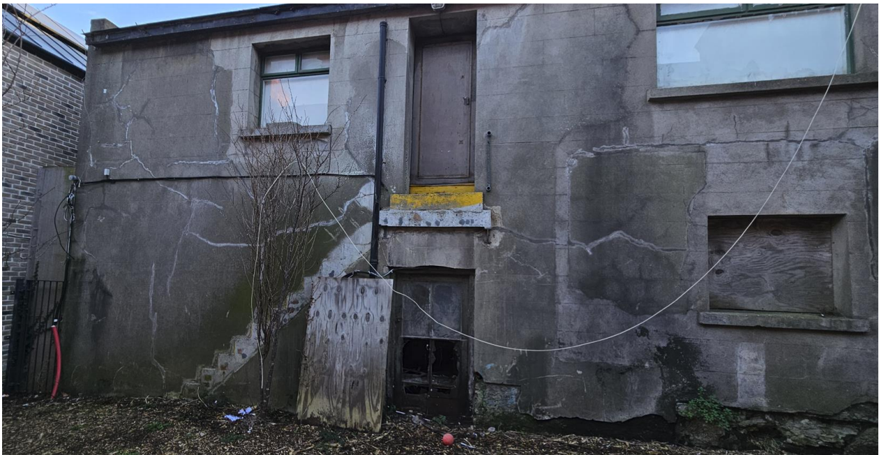
Photo 4. External side view of extension with plywood removed
