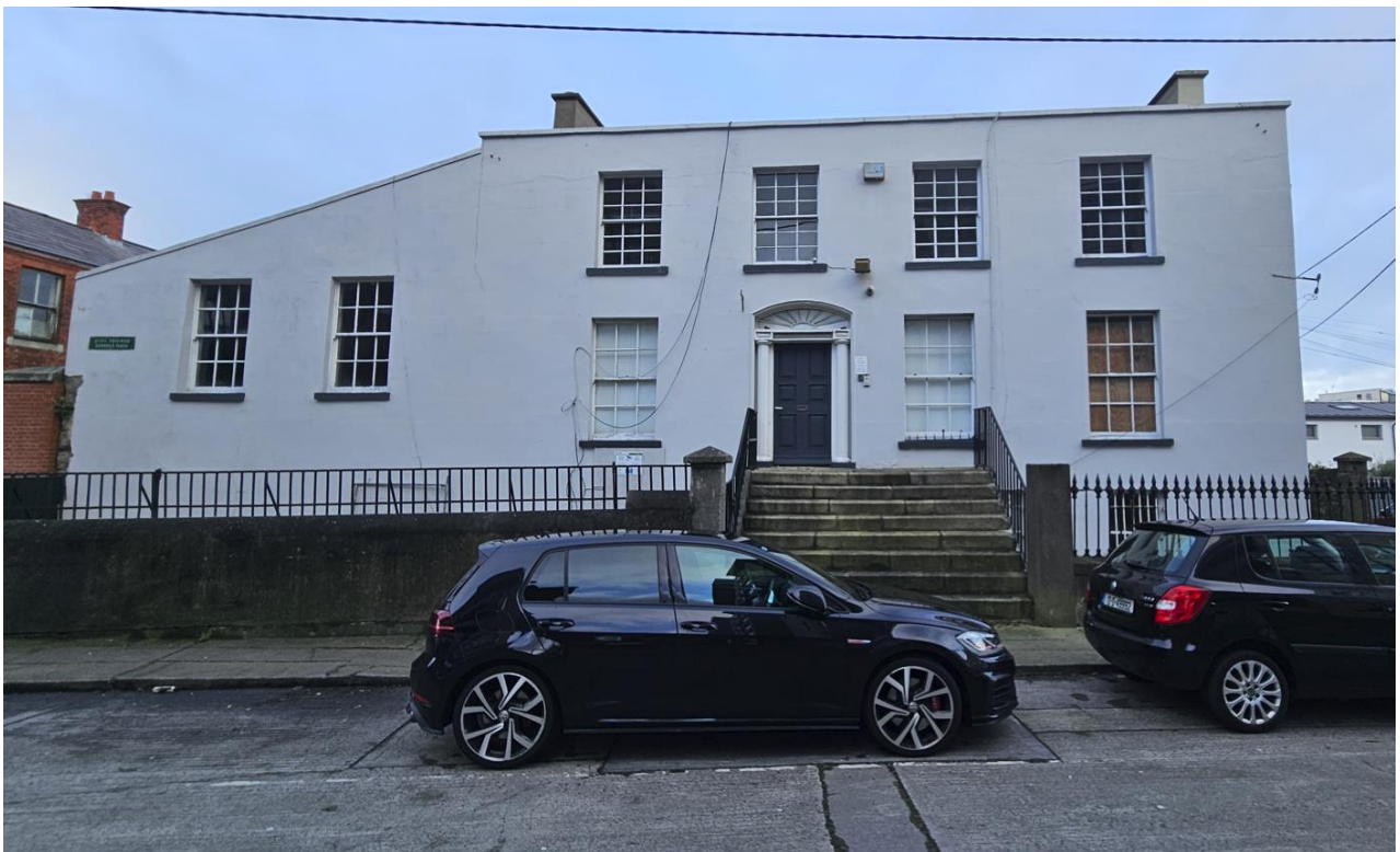
Figure 2: Photo of existing building (No. 9 Georges Place)
