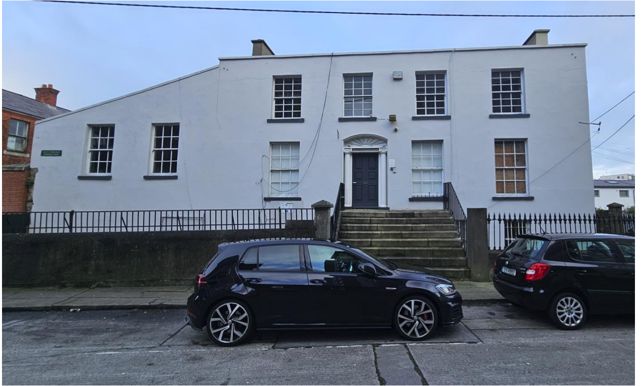
Image 1. View of front facade of No. 9 (south-west facing)
