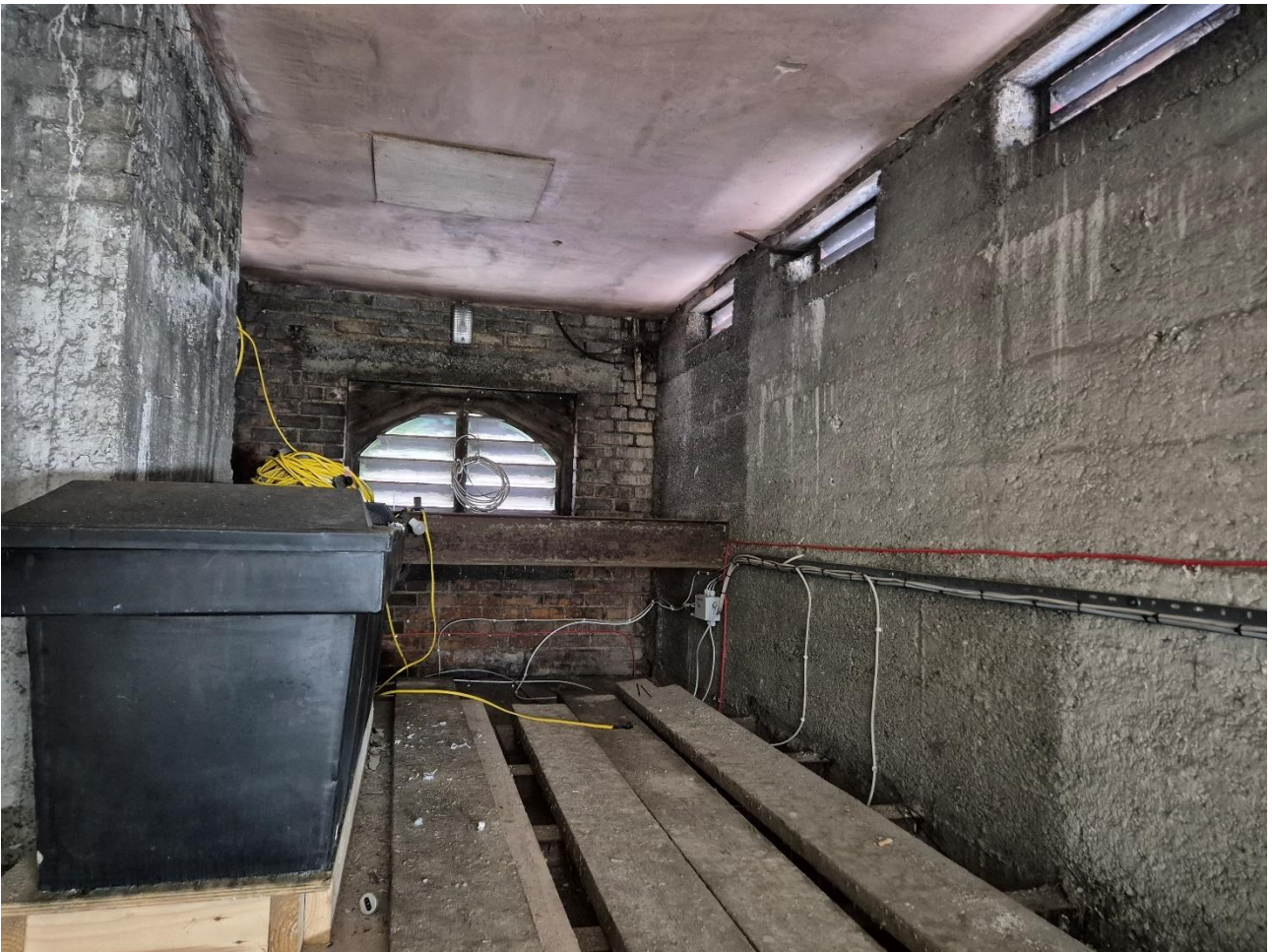
Plate 6: Internal roof room of Wash House, Kellys Avenue, Dún Laoghaire, Co. Dublin depicting side vents (open) and louver window (steel mesh externally).
