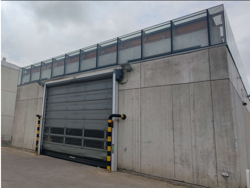
Figure 4 - Existing Unfit for Purpose Salt Barn
