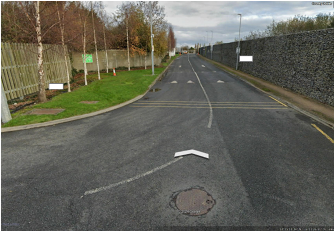
Figure 3-3: Gabion wall on western site boundary at location of proposed new entrance
