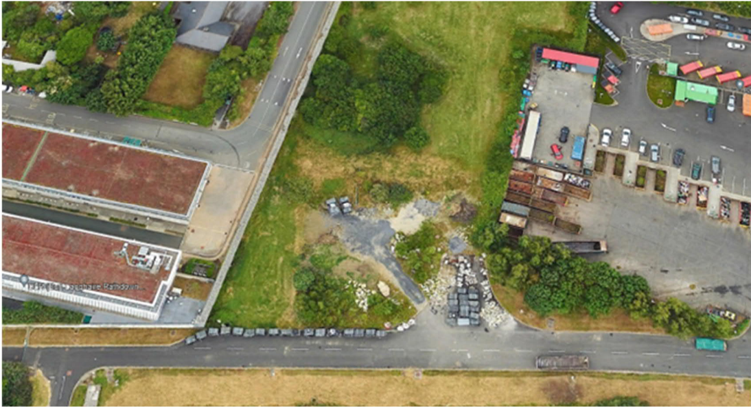
Figure 3-2: Aerial view of existing site (Source: Google Earth)
