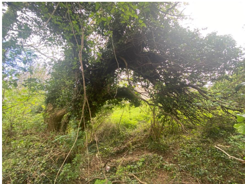
Figure 3.11 Tree densely covered with ivy (>5cm thick) located south of the Site across the private industrial road – photo taken 16/04/2024.
