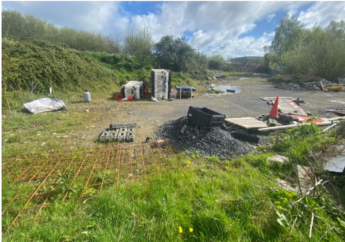
Figure B.7 Recolonising Bare Ground (ED3, as per Fossitt, 2000) – photo taken 16/04/2024
