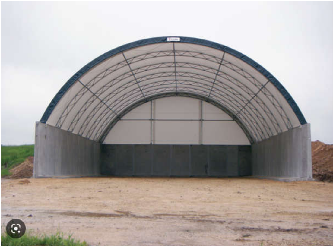
Figure 5 – Example of a Purpose Made Salt Barn
