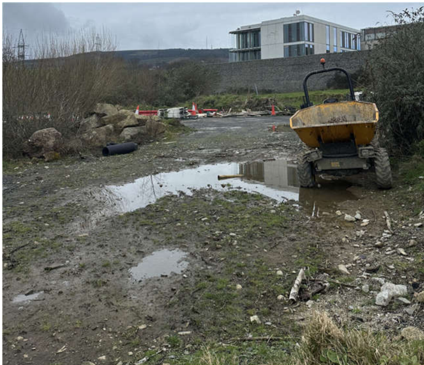
Figure 3-1 Spoil and Bare Ground (ED2, as per Fossitt, 2000).
