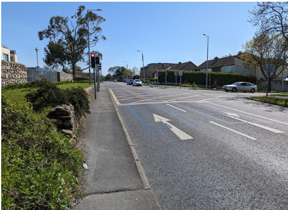
Figure 21 Existing condition at Rochestown Avenue / Johnstown Road signalised junction
