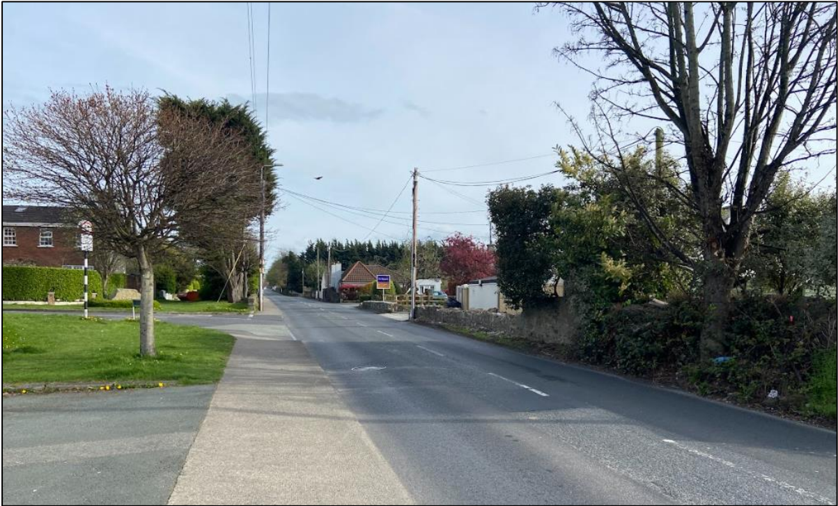
Figure 9 Existing conditions along Rochestown Avenue near Grangewood
