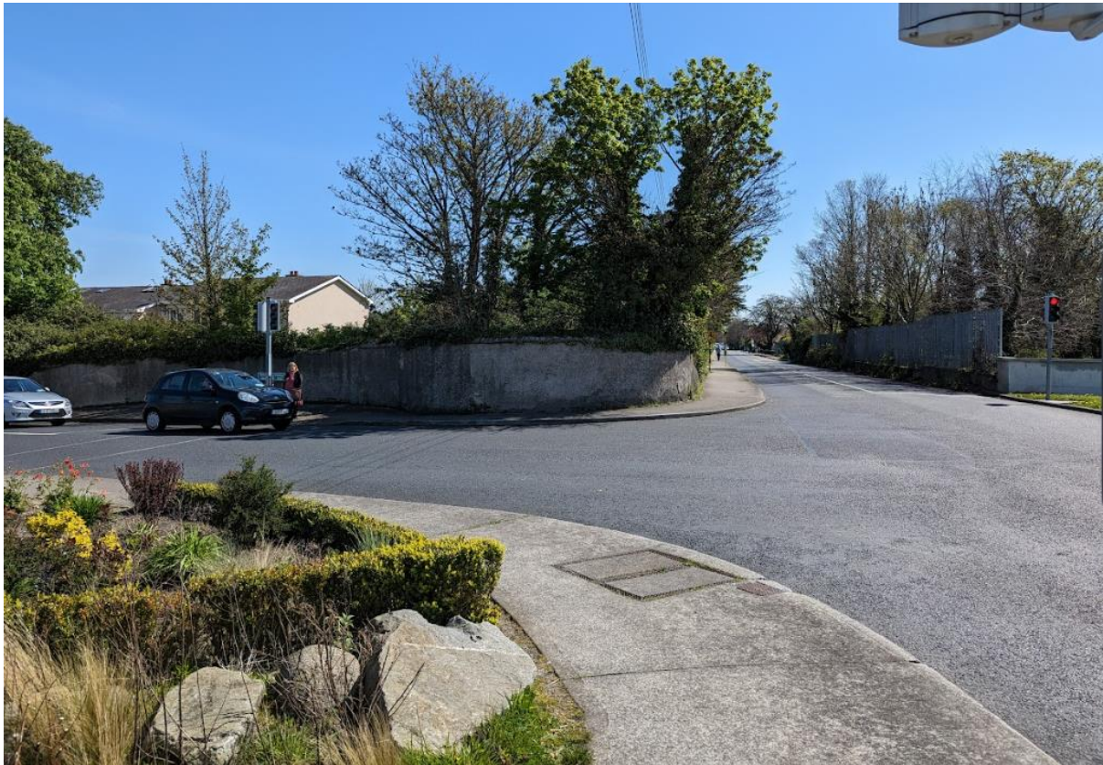
Figure 4-8 Existing Conditions at Rochestown Avenue / Sallynoggin Road junction
