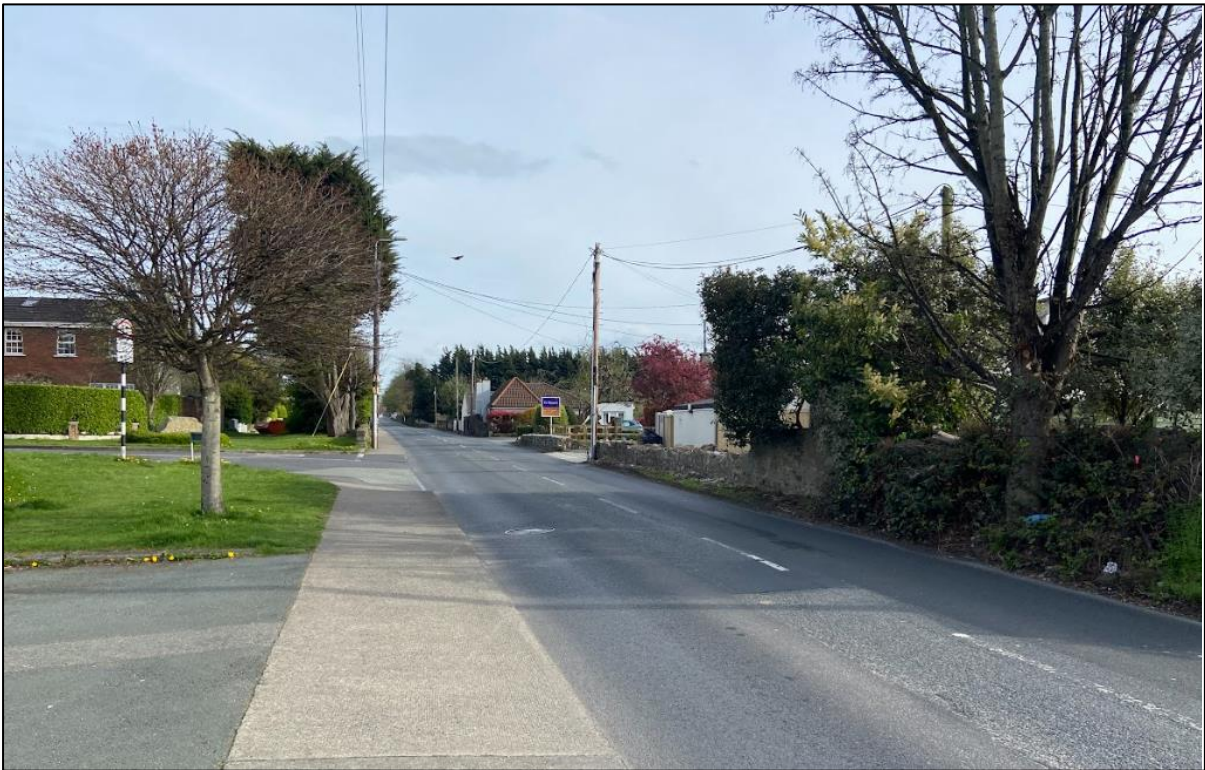
Figure 4-2 Existing conditions along Rochesotwn Avenue near Grangewood
