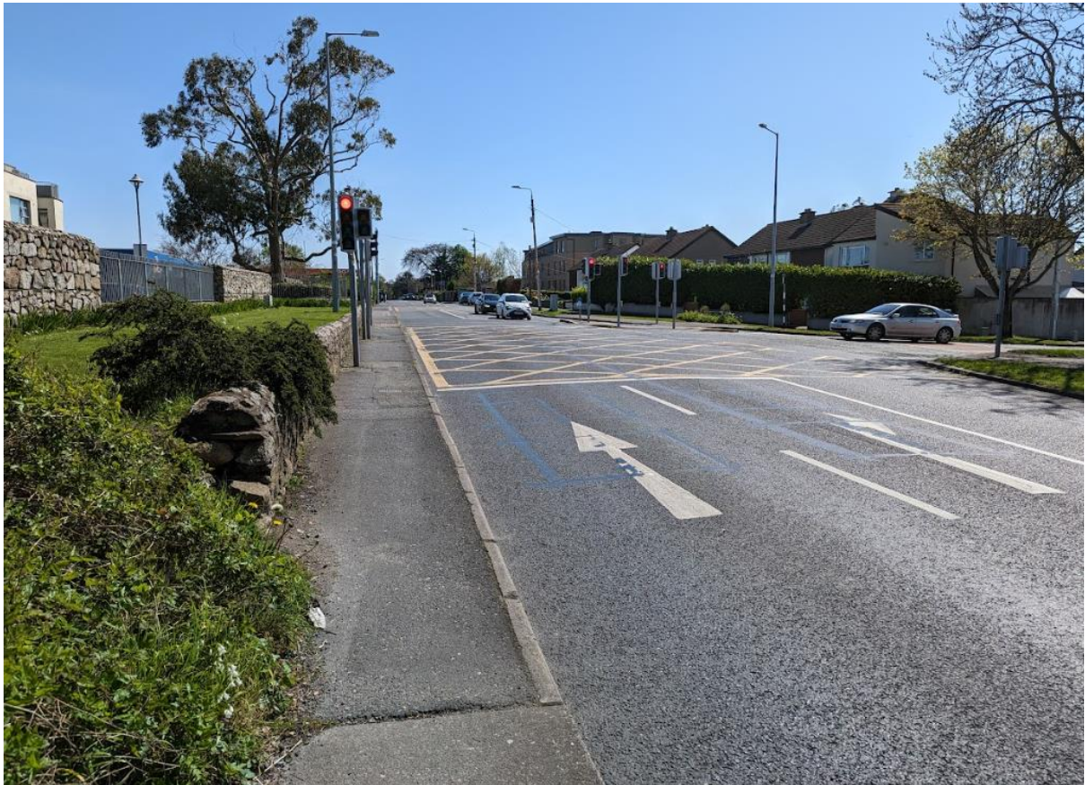
Figure 4-14 Existing condition at Rochestown Avenue / Johnstown Road signalised junction
