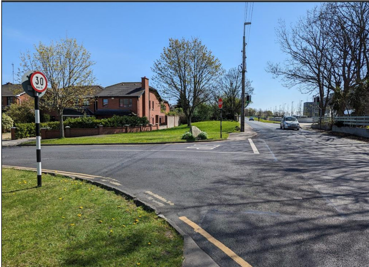
Figure 4-6 Existing Conditions along Rochestown Avenue near Sefton
