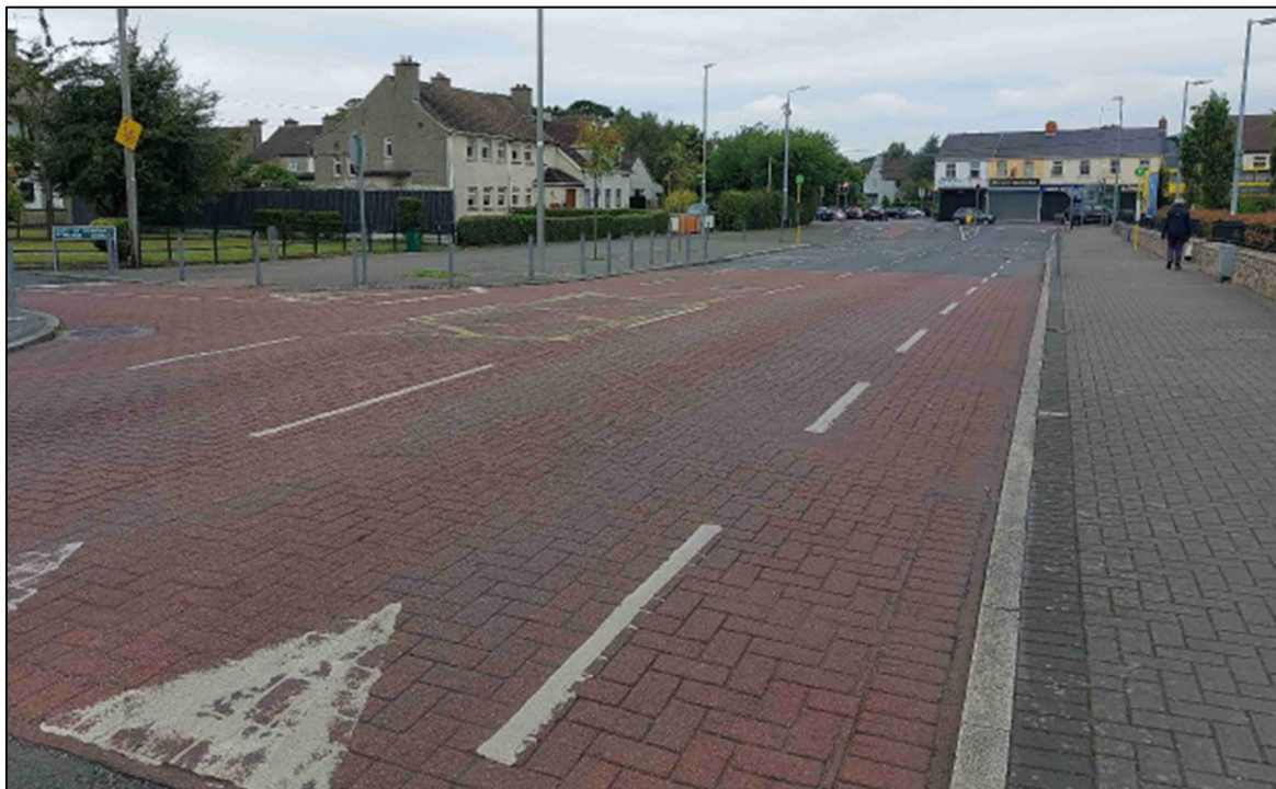
Photograph 1– Pearse St, school side looking west
