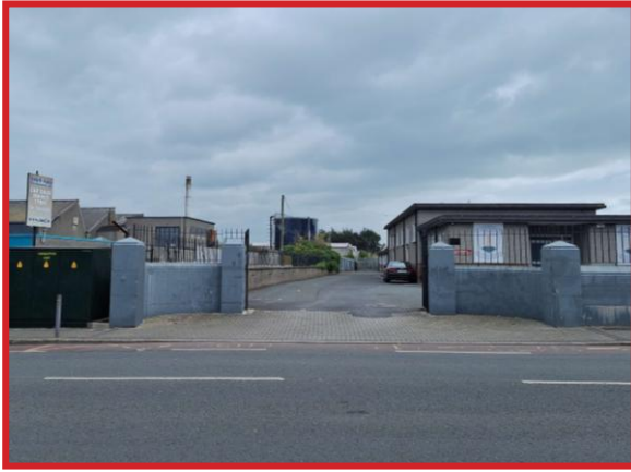
Existing vehicular entrance to St. Kevin's NS on Pearse Street
