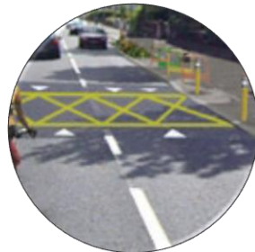
Raised pedestrian crossing
