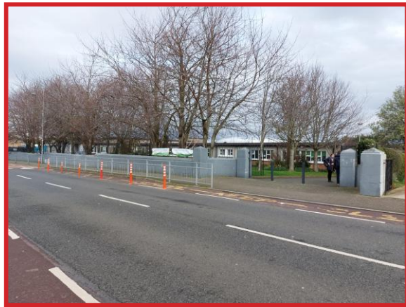
Existing pedestrian entrance to St. Kevin's NS on Pearse Street
