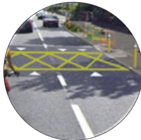
Raised pedestrian crossing
