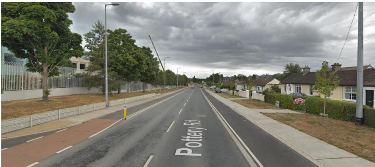
Figure 7-1 Example one-way kerb protected cycle track
