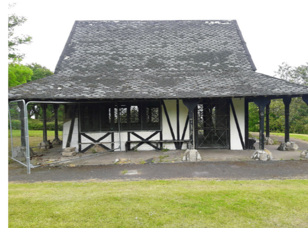
View of disused kiosk pavilion
