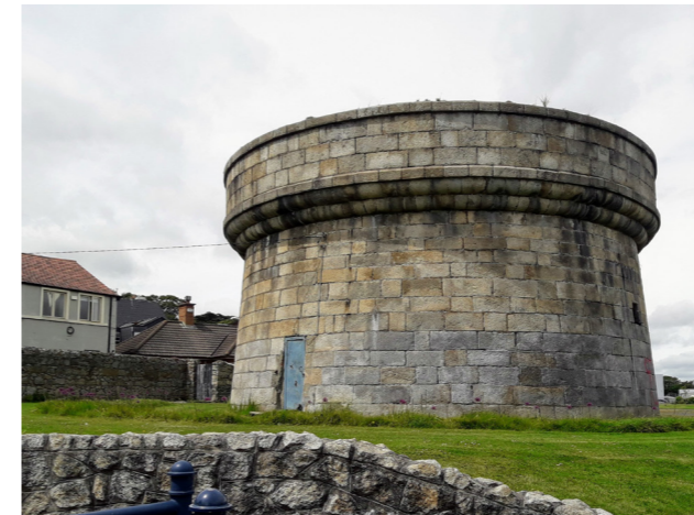
View of the disused Martello Tower
