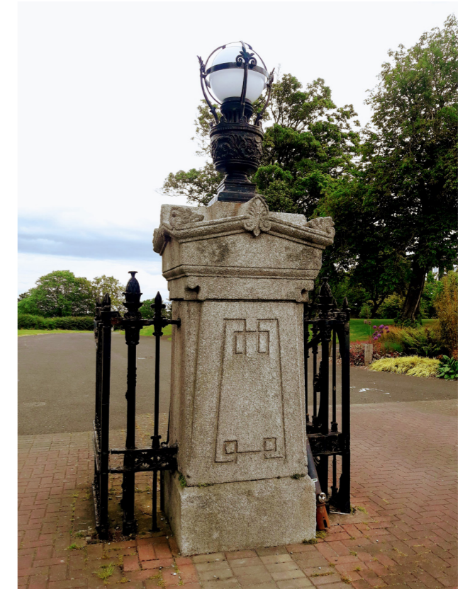
View of granite piers featuring Beux Arts details
