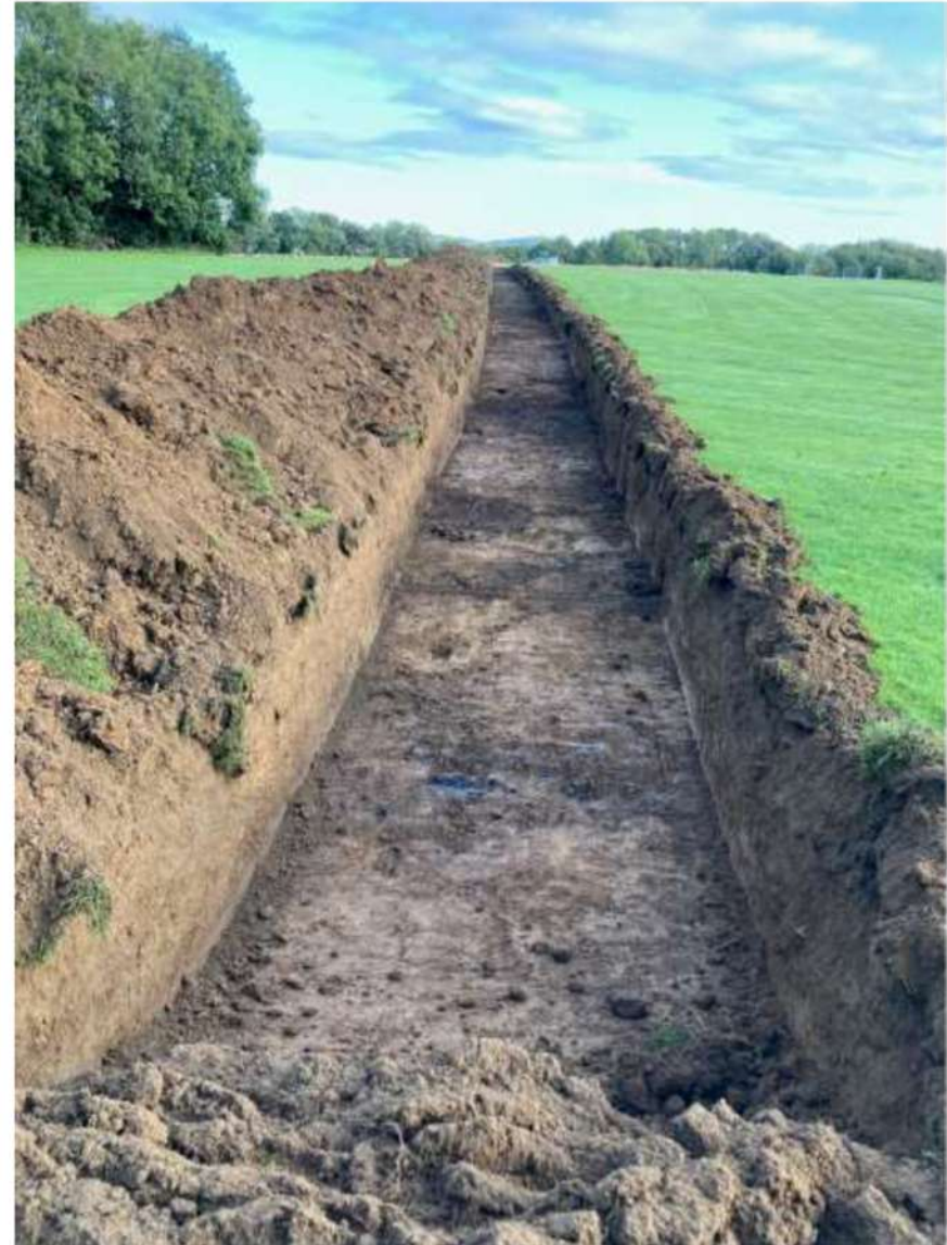
Plate 61: Test trench 24, facing north
