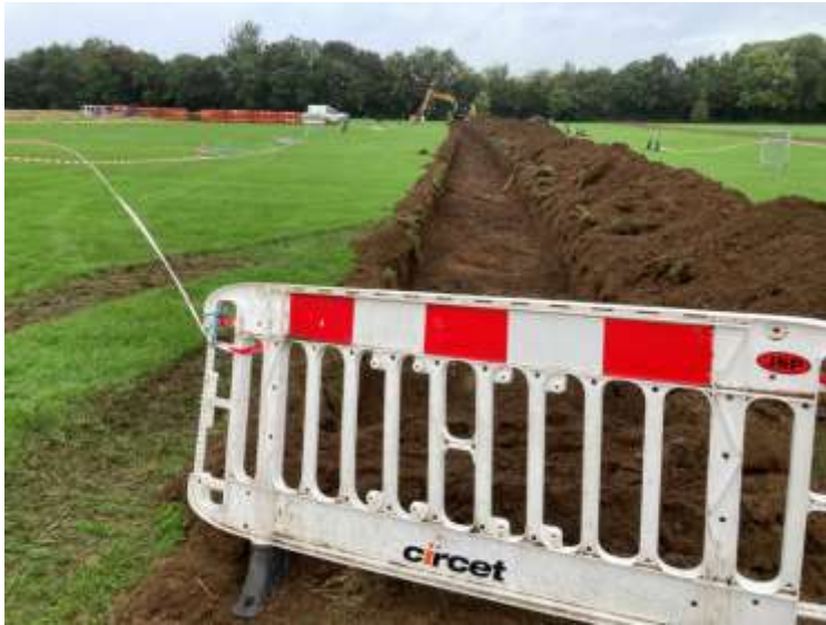
Plate 15: Test trench 4, facing north
