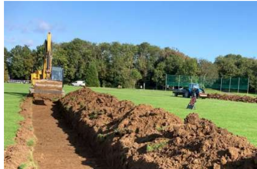
Plate 4: Trenching at baseball terrain, facing north
