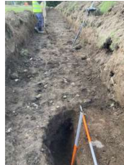
Plate 32: Test trench 11, facing southeast
