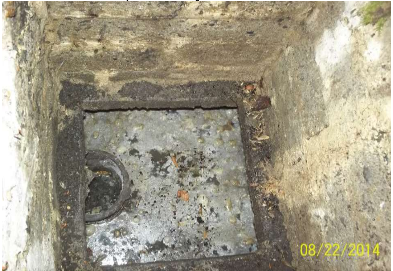
Photos Septic Tank showing inlet T-Piece
