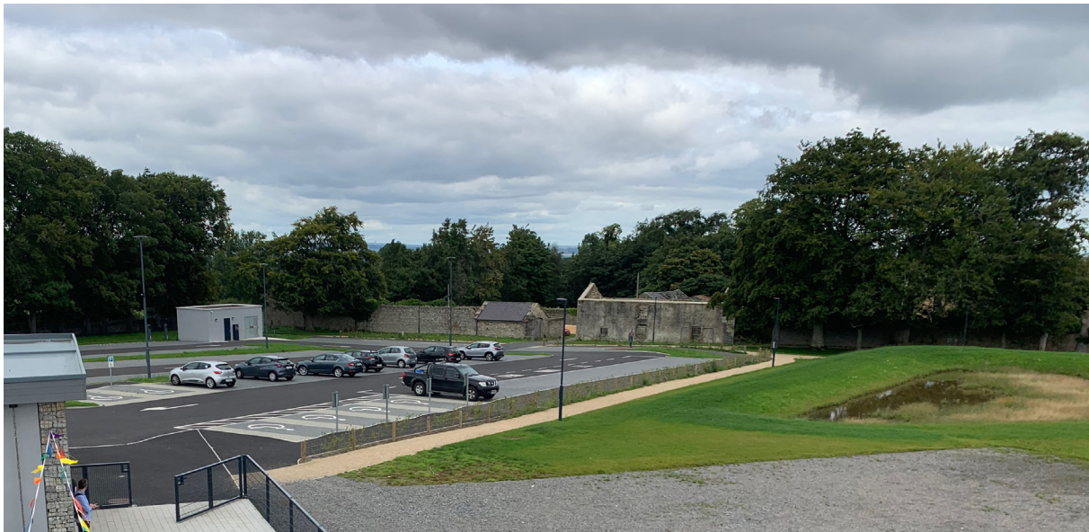
FIGURE 9: ELEVATED VIEW TOWARDS ST THOMAS HOUSE ACROSS THE FRONT OF THE SUBJECT SITE
